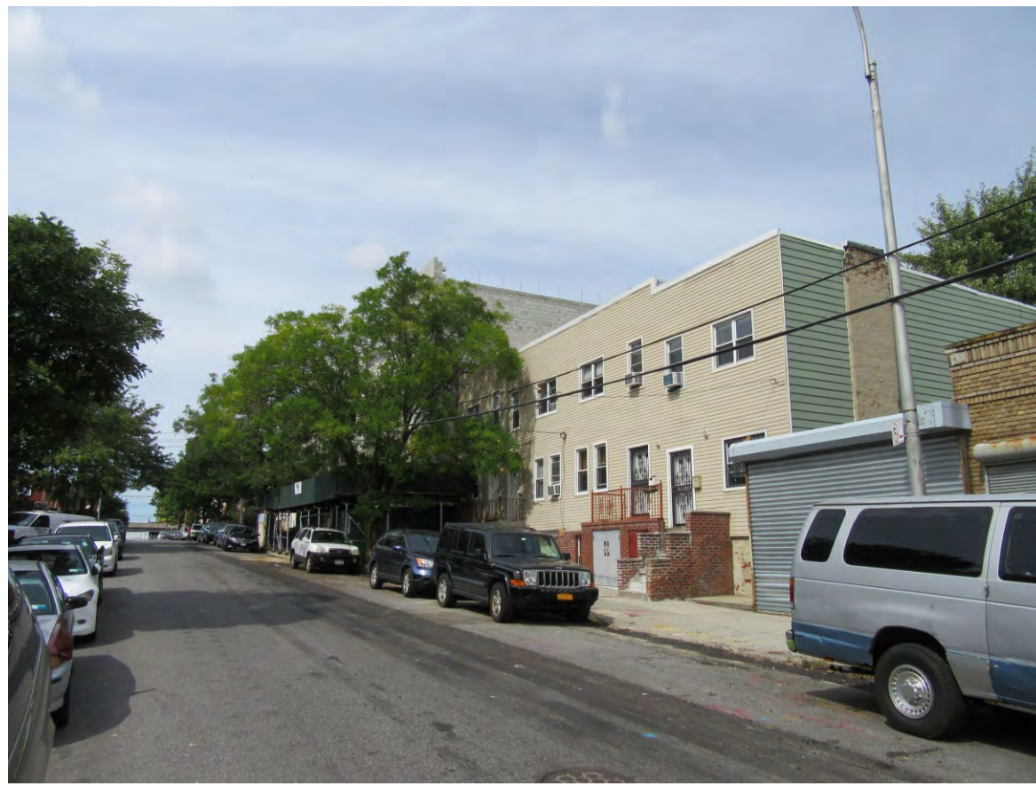
7. View of the north side of East 133rd Street between Cypress Avenue and Willow Avenue facing northwest.
