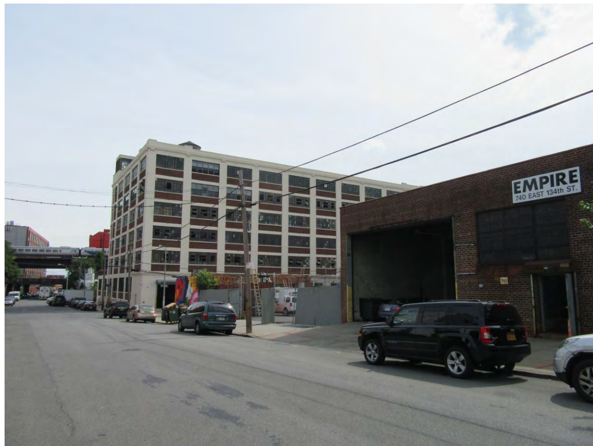
16. View of the Site facing south from East 134th Street.
