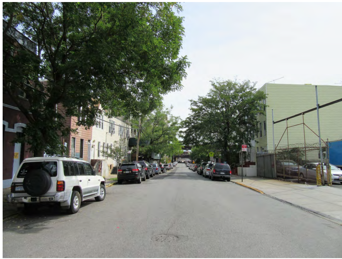
10. View of East 133rd Street between Cypress Avenue and Willow Avenue facing southeast.
