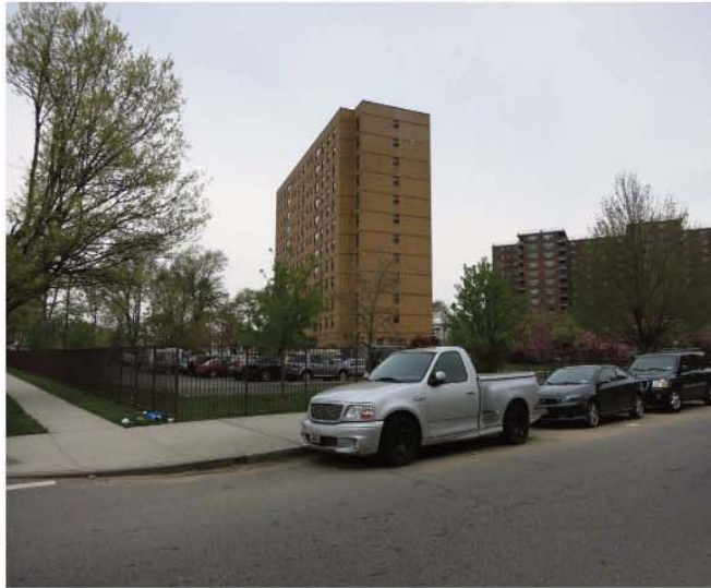
6. View of the Site facing north from the intersection of 132nd Avenue and 161st Street.
