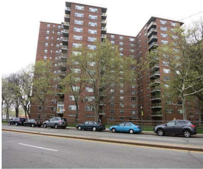
22. View of Guy R Brewer Boulevard facing northeast from the Site.
