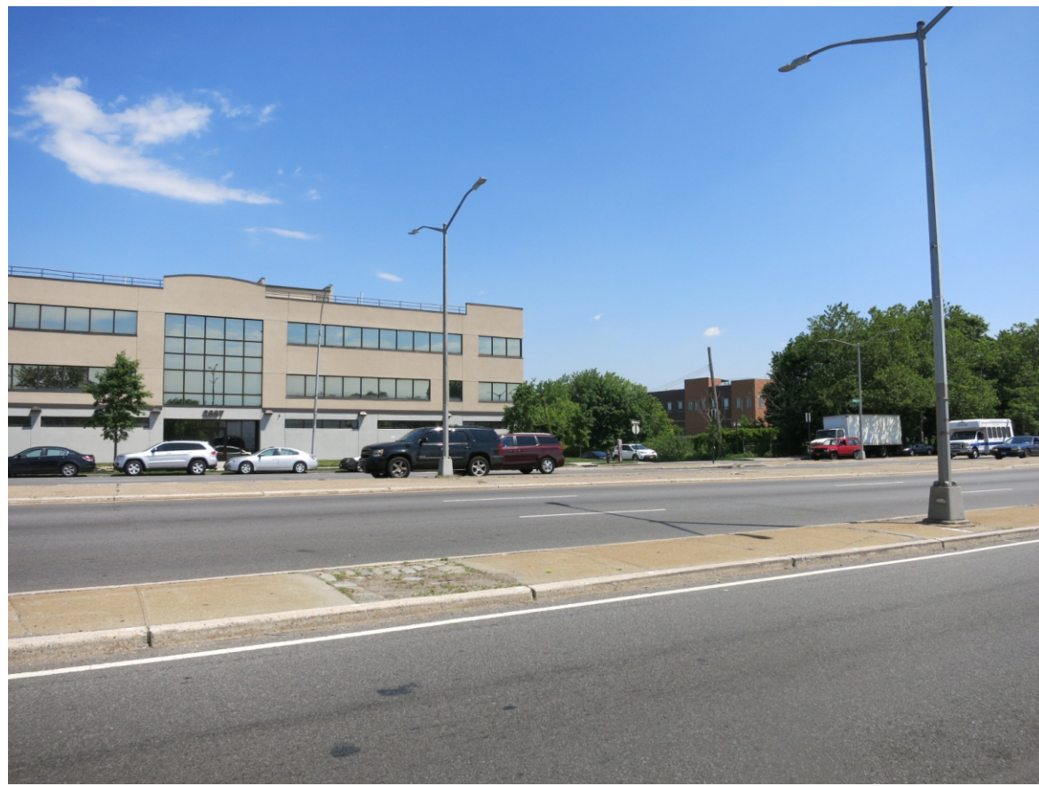
28. View of the side of Linden Boulevard facing northeast from the Site.
