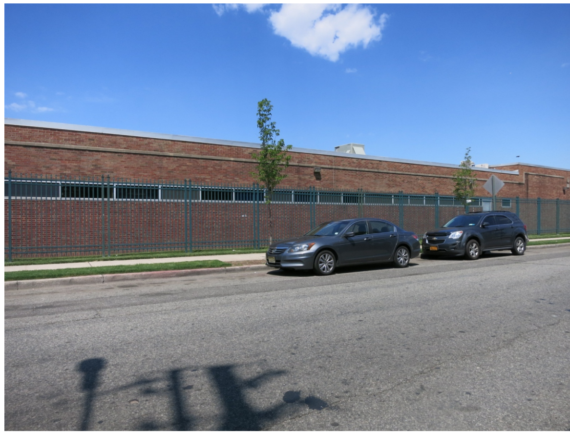
34. View of the side of Emerald Street facing northwest from the Site.
