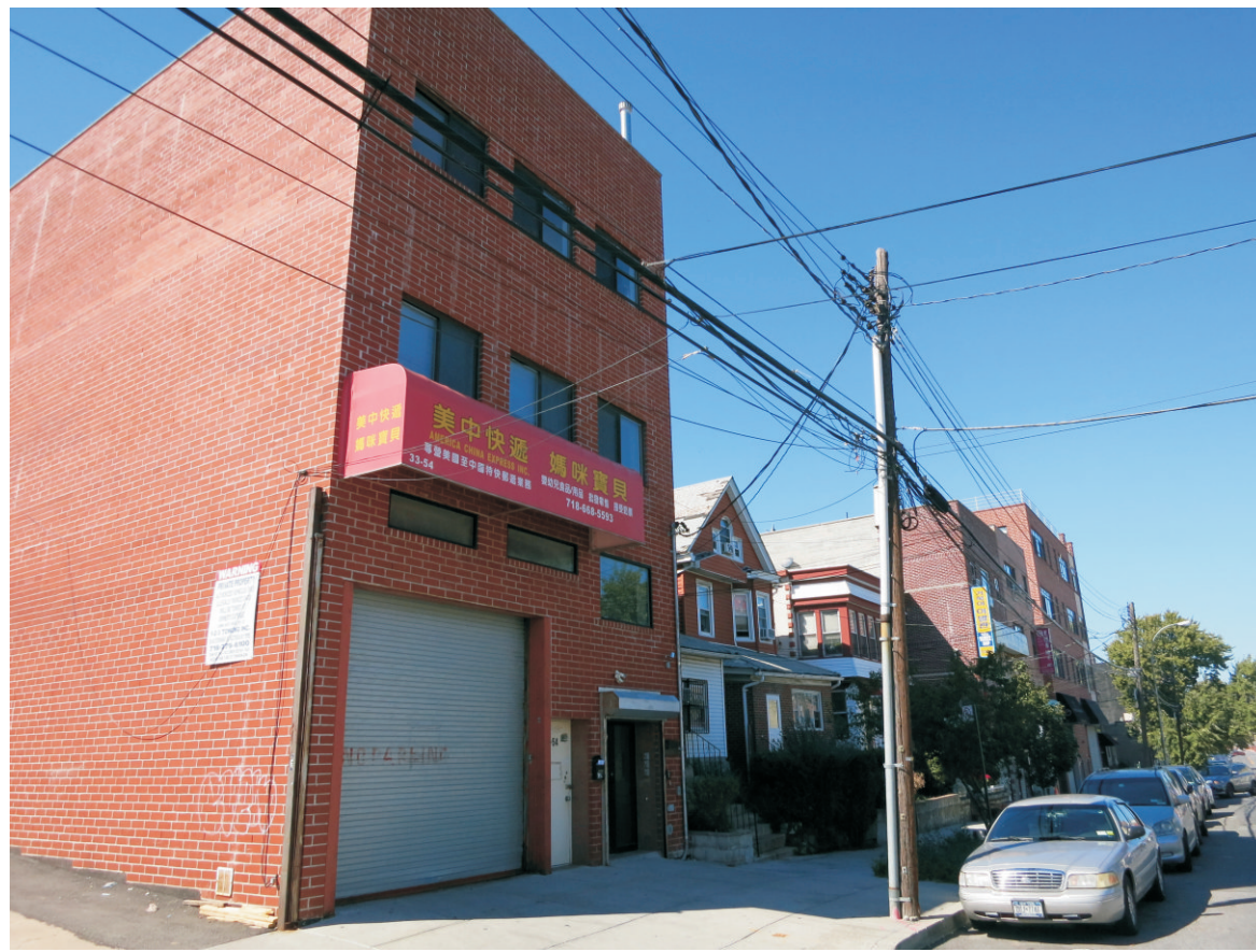
16. View of the side of Farrington Street facing northwest.
