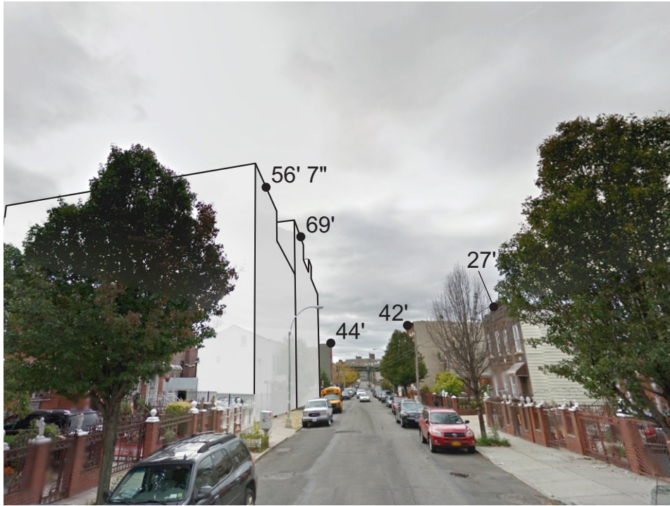
Suydam Street facing southwest (Site at left)
