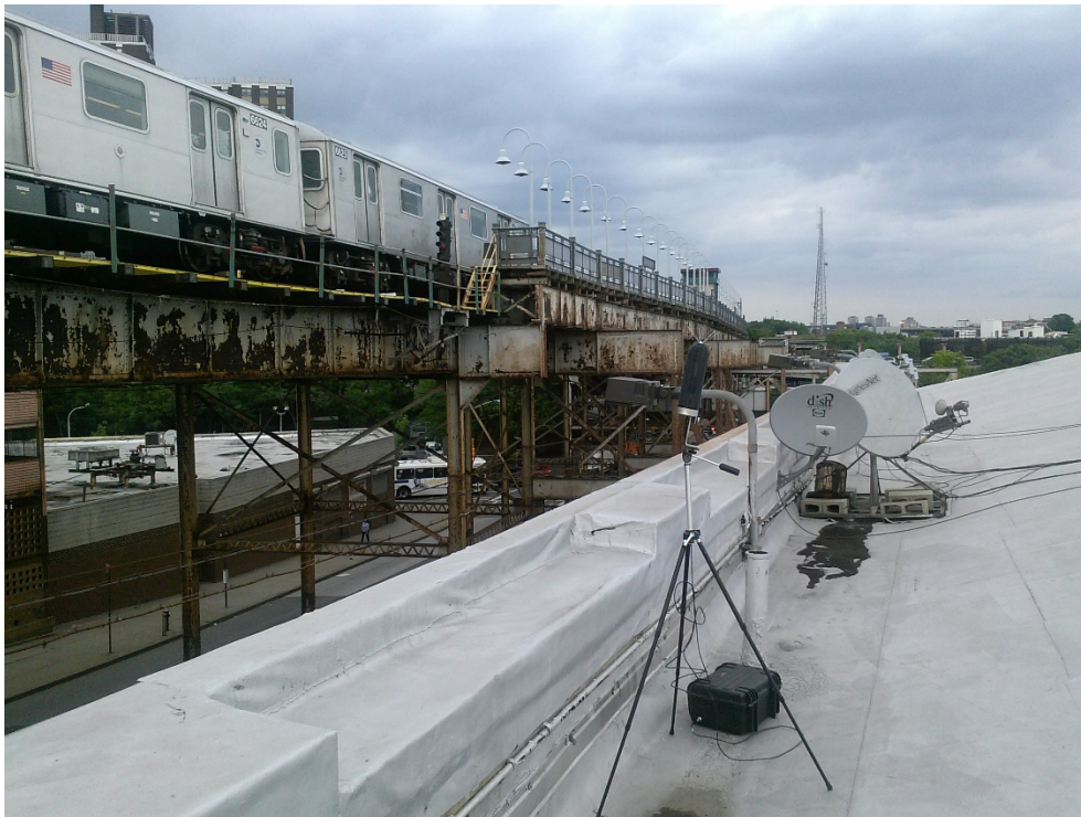
Photo 2: Rooftop noise monitoring location; direction facing: East
