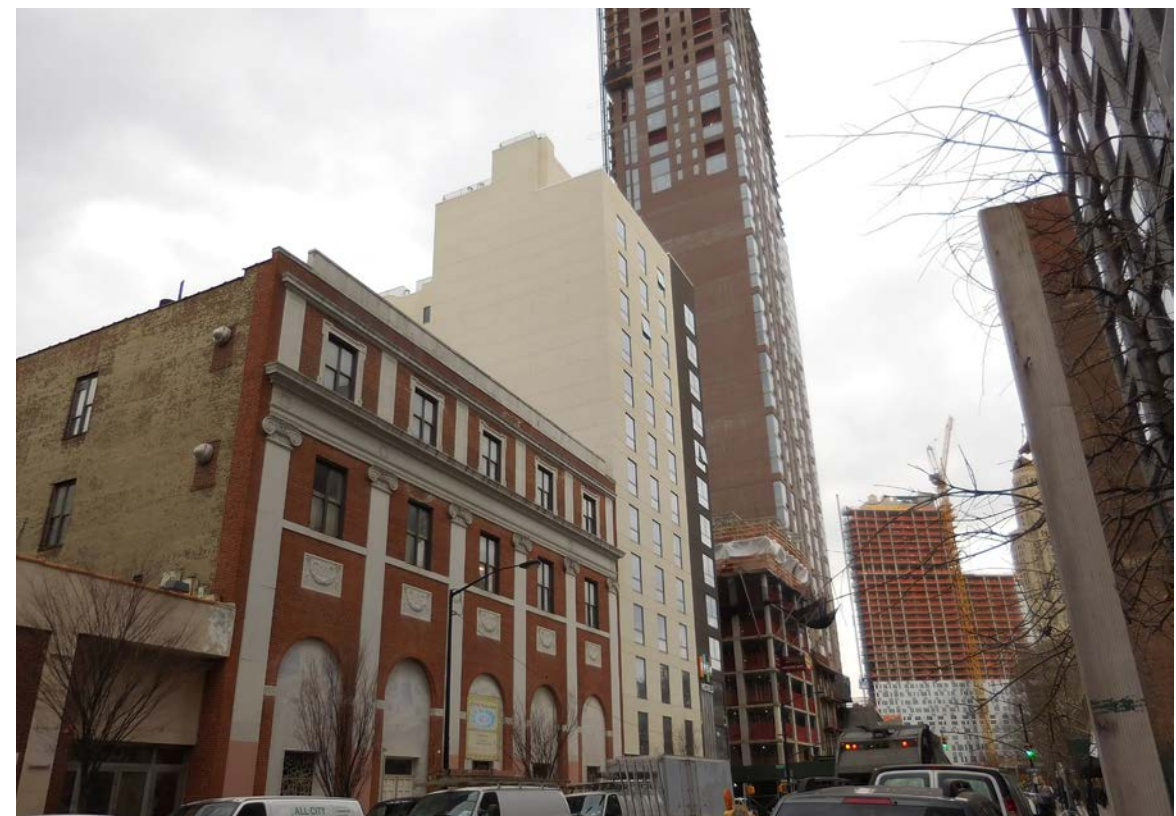
2. View East along Schermerhorn Street. Foreground shows a Hare Krishna Center, and an Even Hotels beyond. Photograph taken on : 02/10/2016
