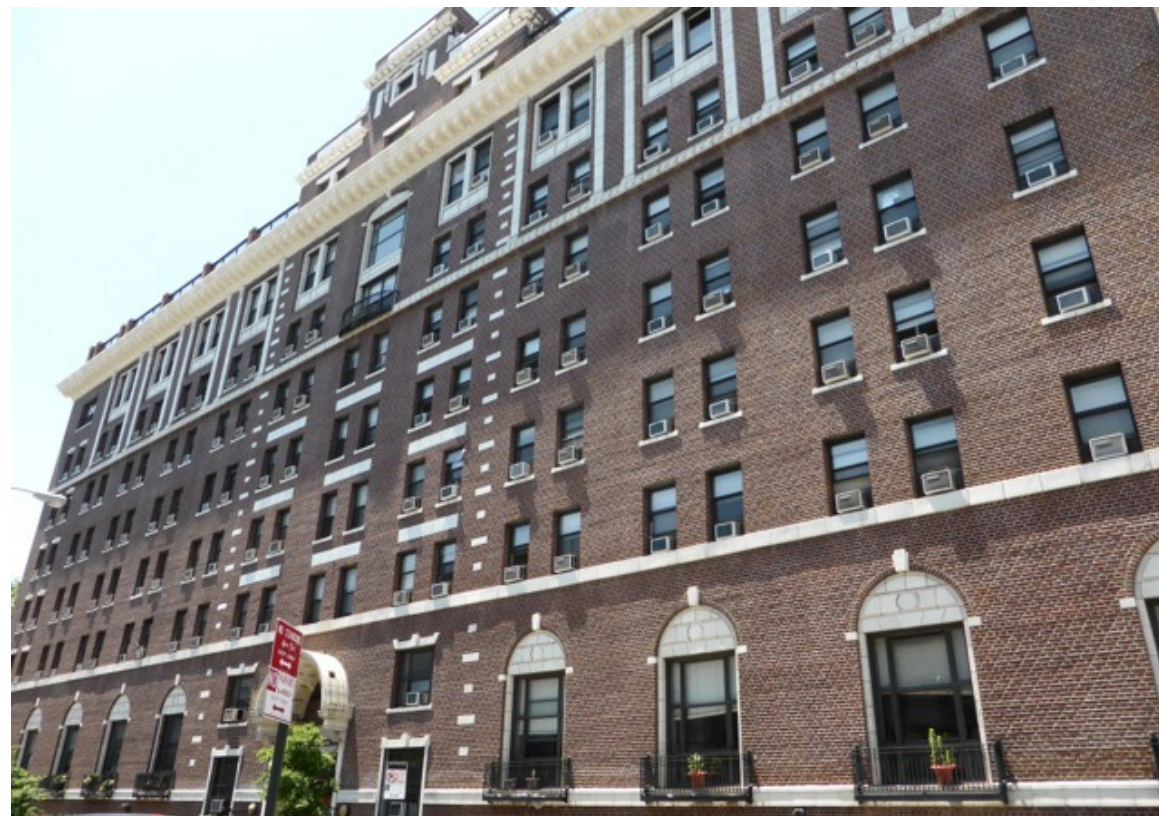
1. View West of East side of building from Nevins Street. Photograph taken on: 04/18/2014
