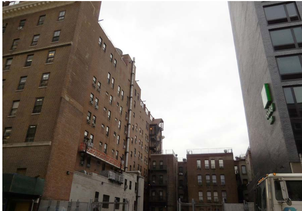
1. View South of West side of building from Schermerhorn St. Photograph taken on: 02/10/2016
