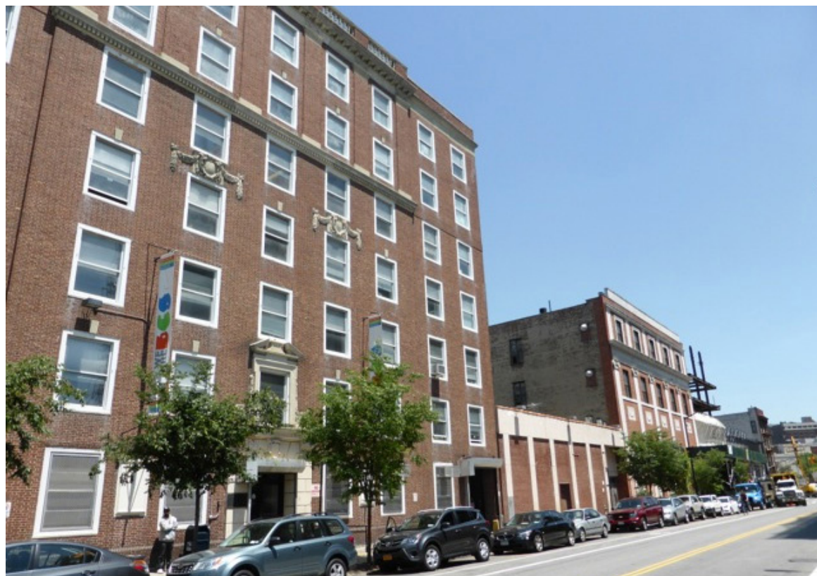
3. View East along Schermerhorn Street. Foreground shows a 7-story residential building. Photograph taken on: 06/18/2014
