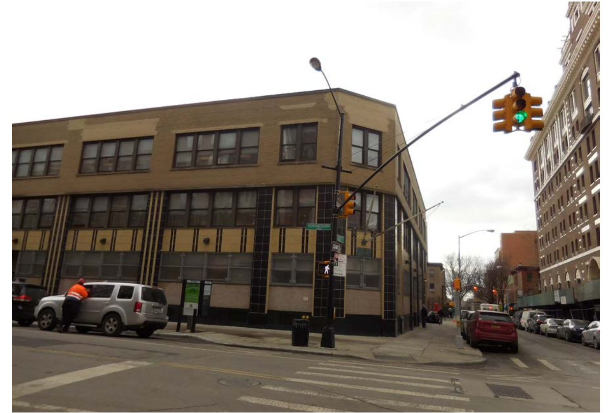
3. View South of Safe Horizon Child Advocacy building, directly opposite of project area. Photograph taken on: 02/10/2016
