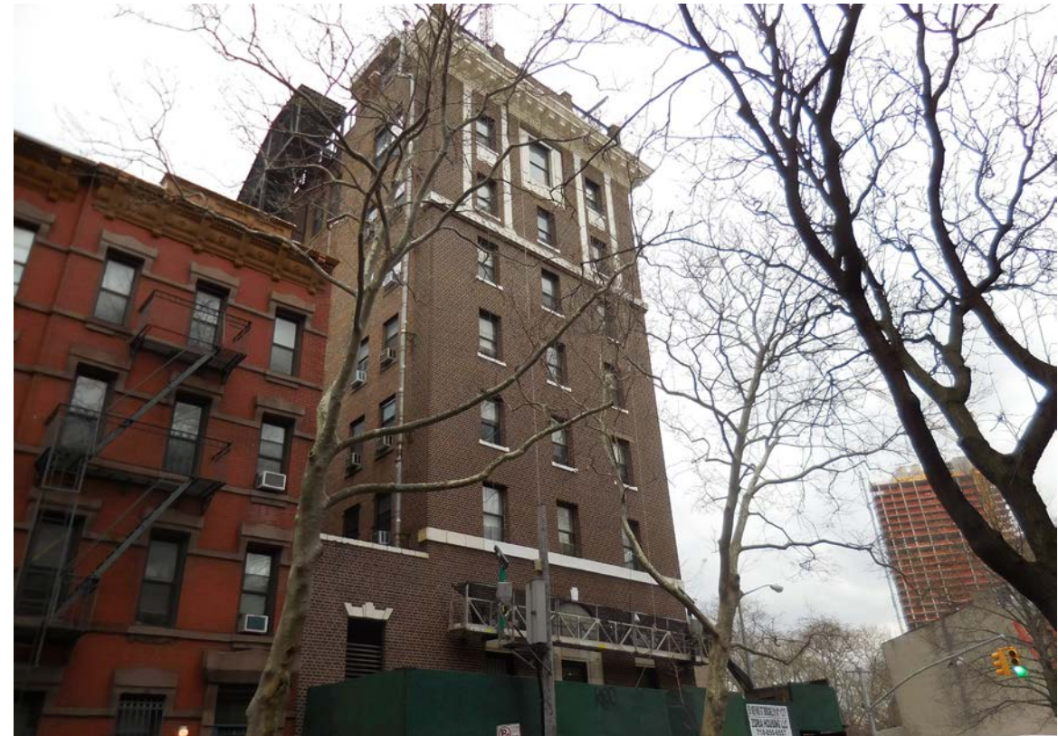
2. View East of South side of building from State Street. Photograph taken on: 02/10/2016
