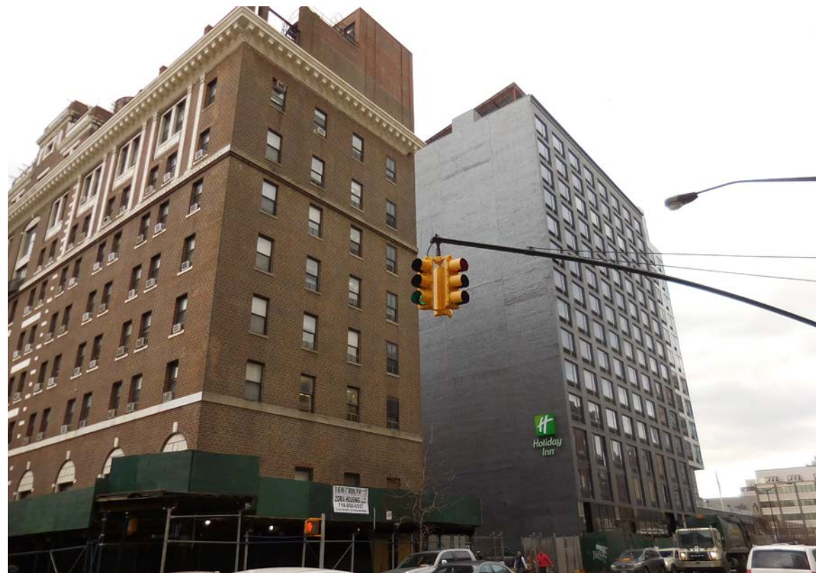
3. Facing E. View of N side of building and adjacent Holiday Inn from corner of Schermerhorn St. and Nevins St. Photograph taken on: 02/10/2016
