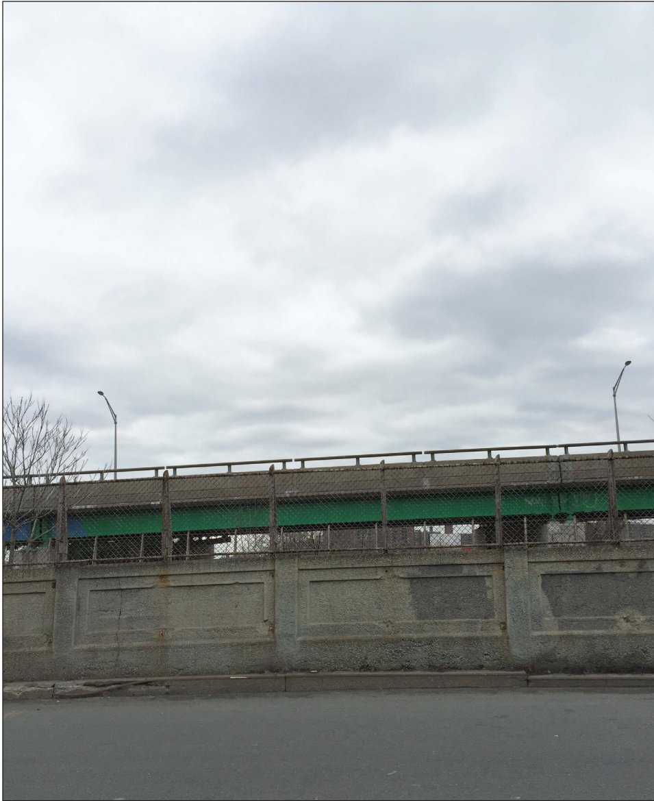
Looking east from the Project Site on Whitlock Avenue
