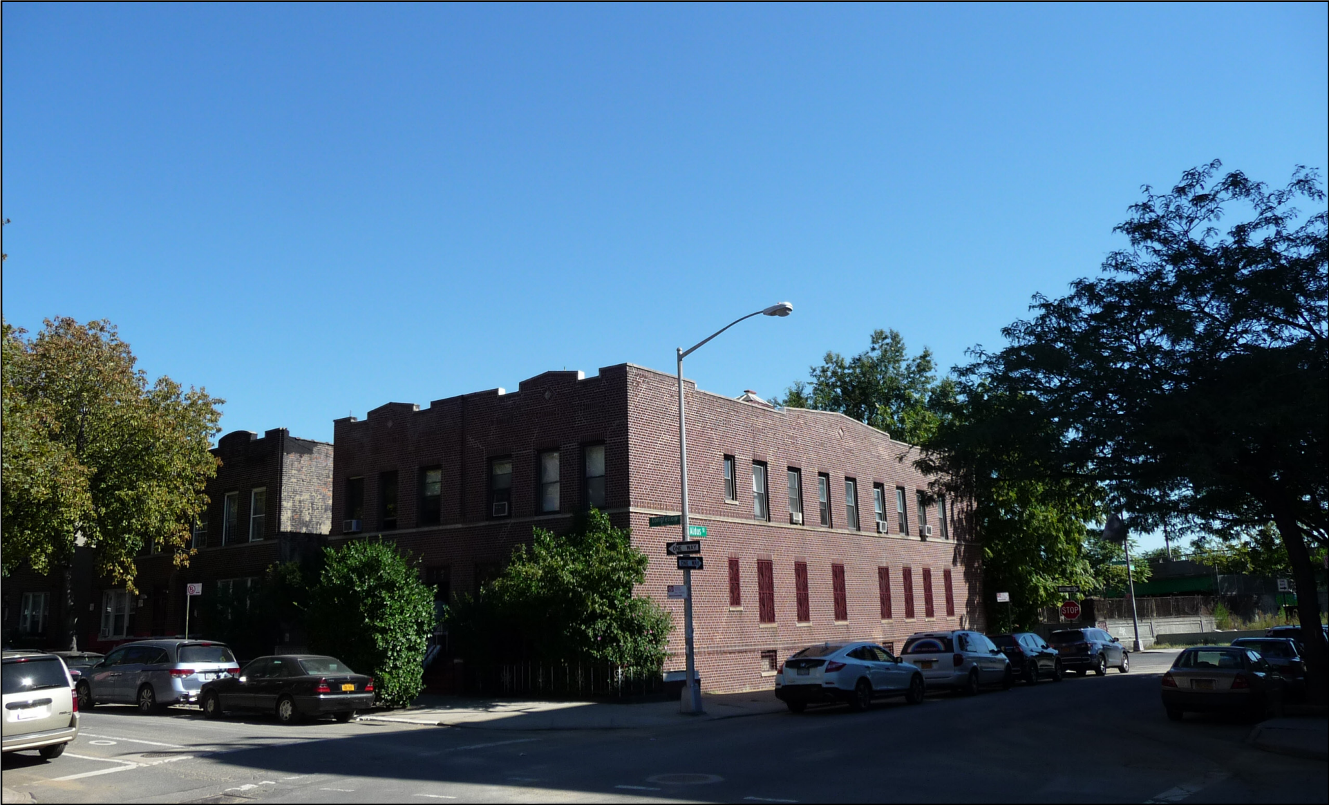
FIGURE 23: TWO-FAMILY HOMES ALONG LONGFELLOW AVENUE Whitlock and 165th Street Rezoning
