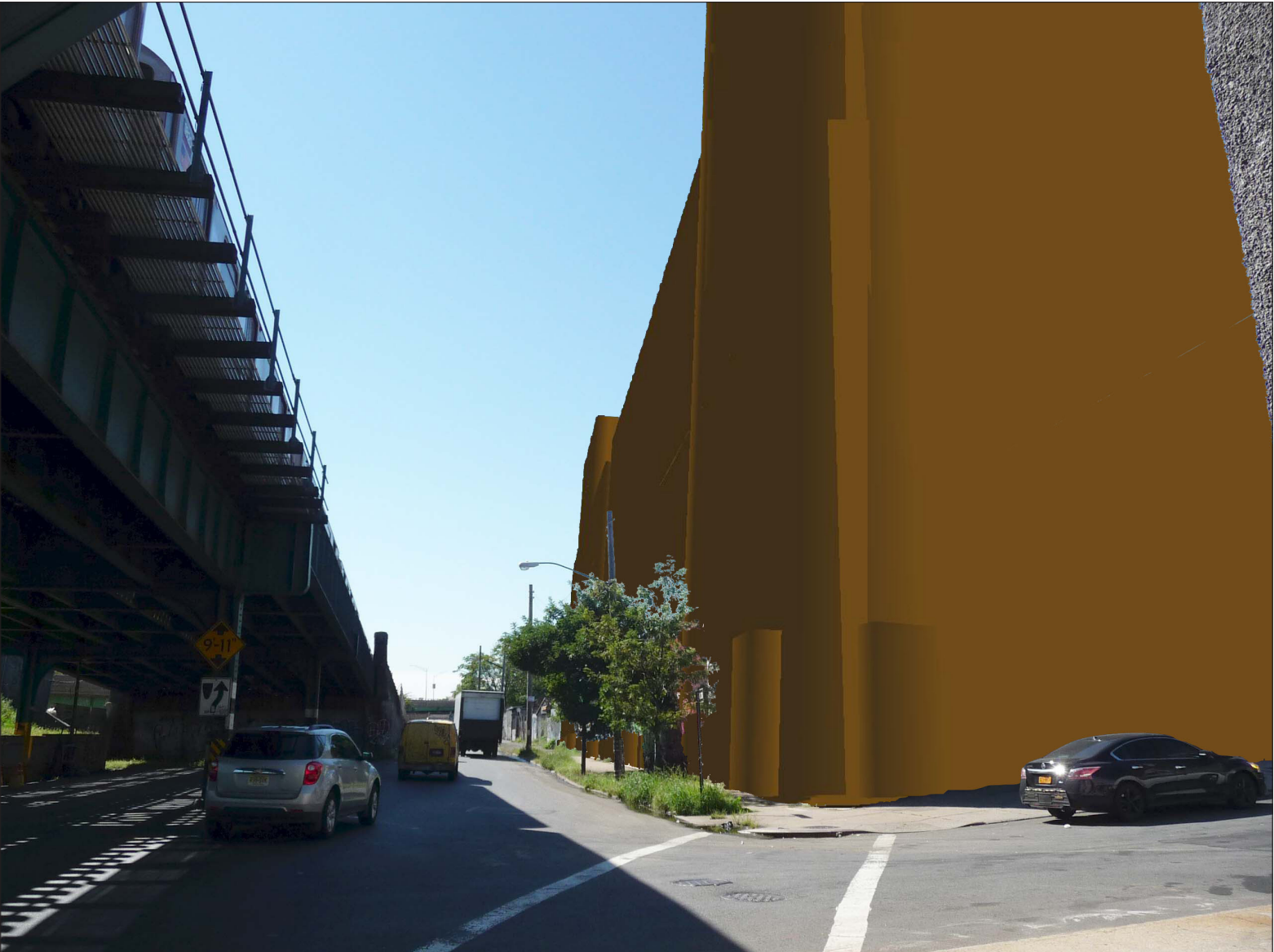
View 1: Looking south on Whitlock Avenue at the intersection of East 165th Street and Whitlock Avenue
