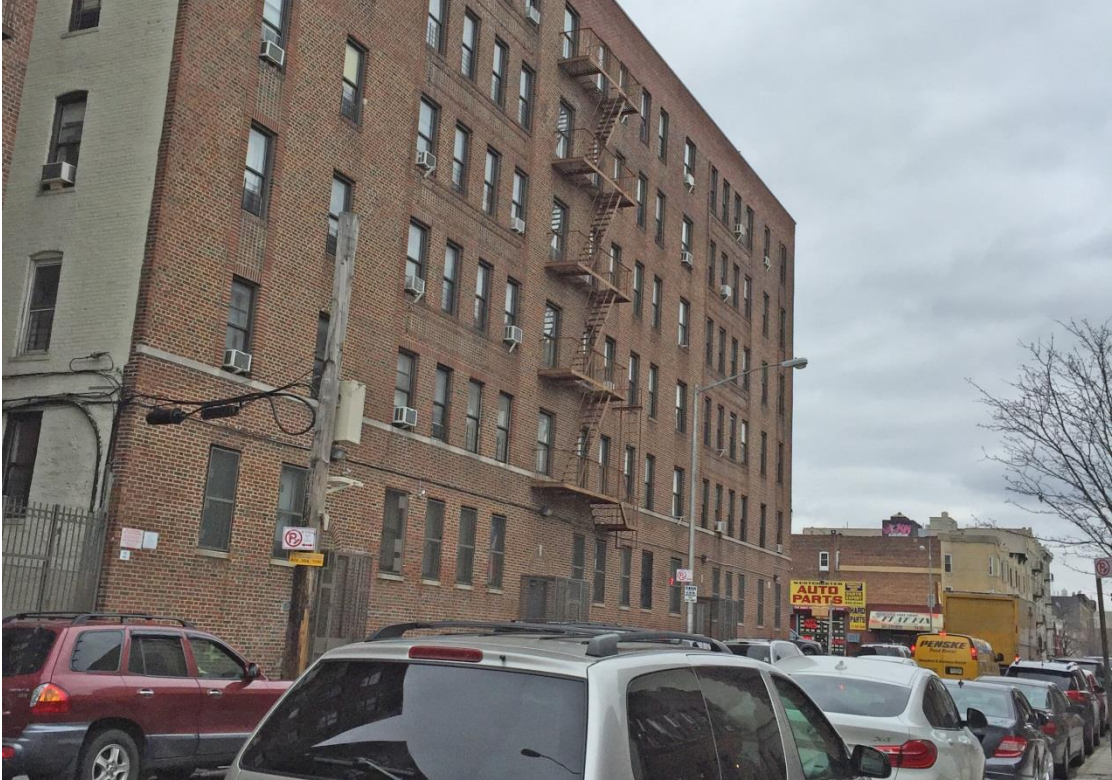
Photograph 11: Northwest view of residential buildings from Lowell Street
