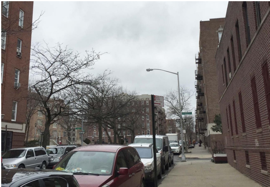
Photograph 6: West view of residential buildings along Aldus Street from Project Site
