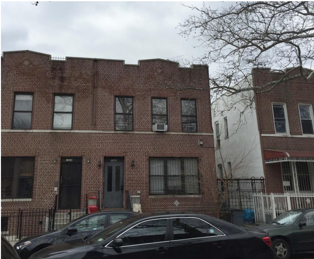
Photograph 14: East view towards Project Site of residences along Longfellow Avenue (central block)
