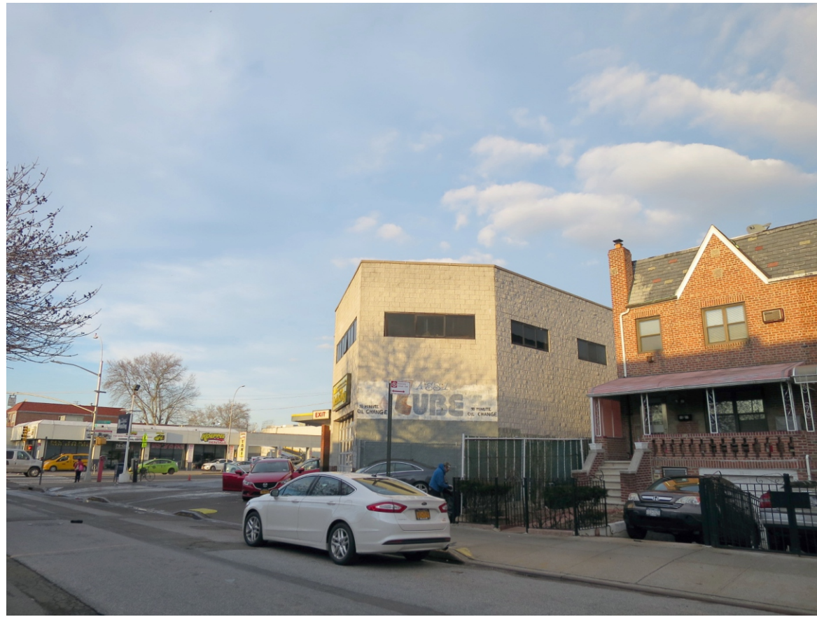
1. View of the Site facing northeast from 74th Street.
