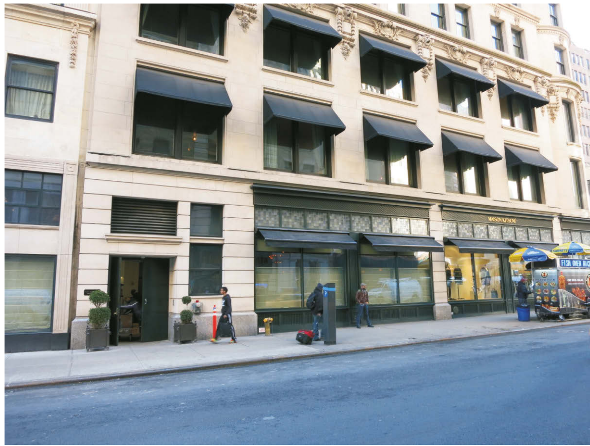
10. View of the Site facing southwest from West 28th Street.
