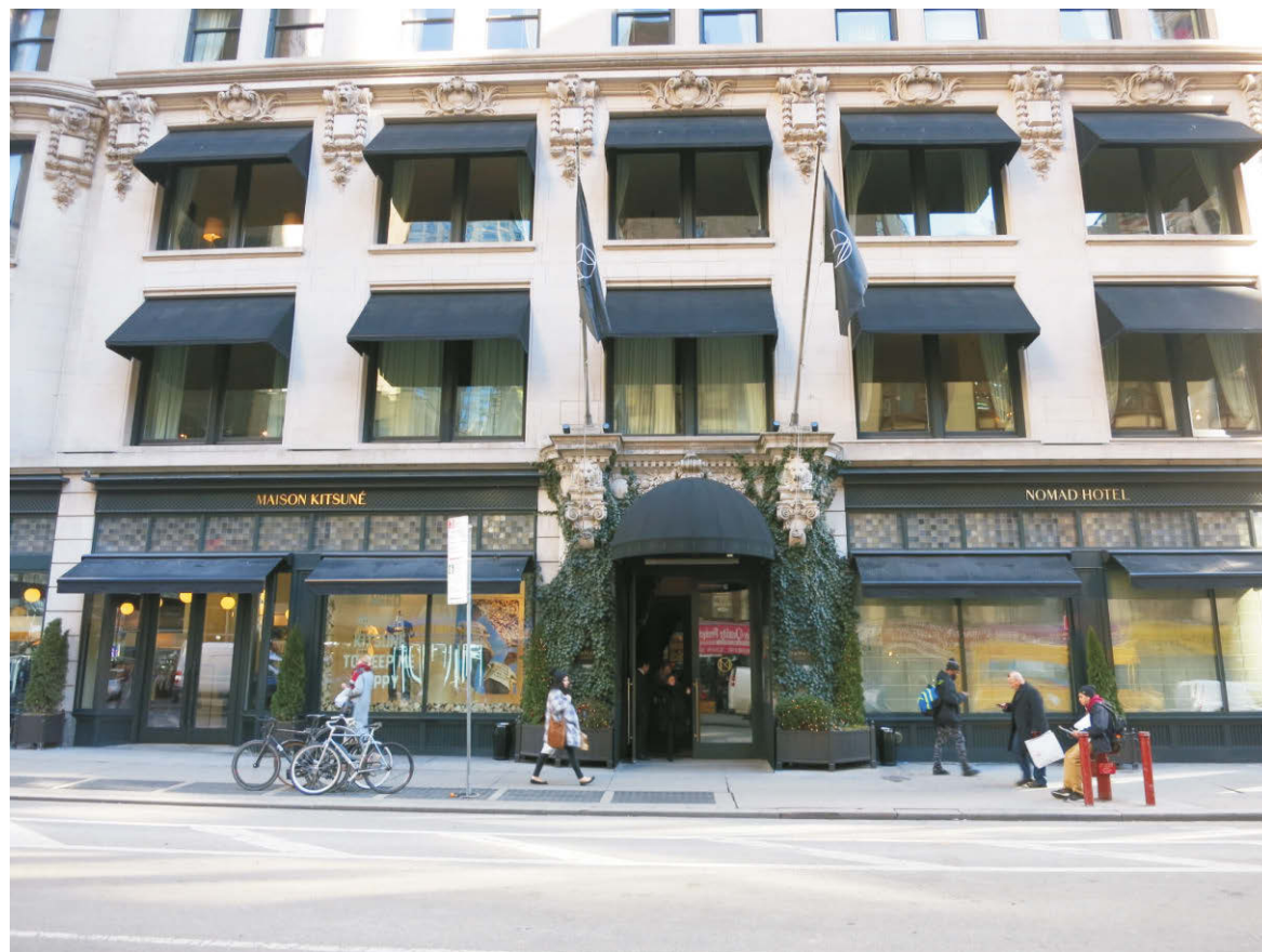
3. View of the Site facing east from Broadway.
