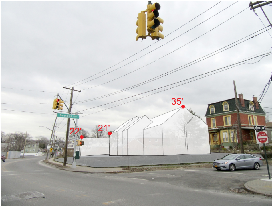
Richmond Terrace facing east (Site at right)
