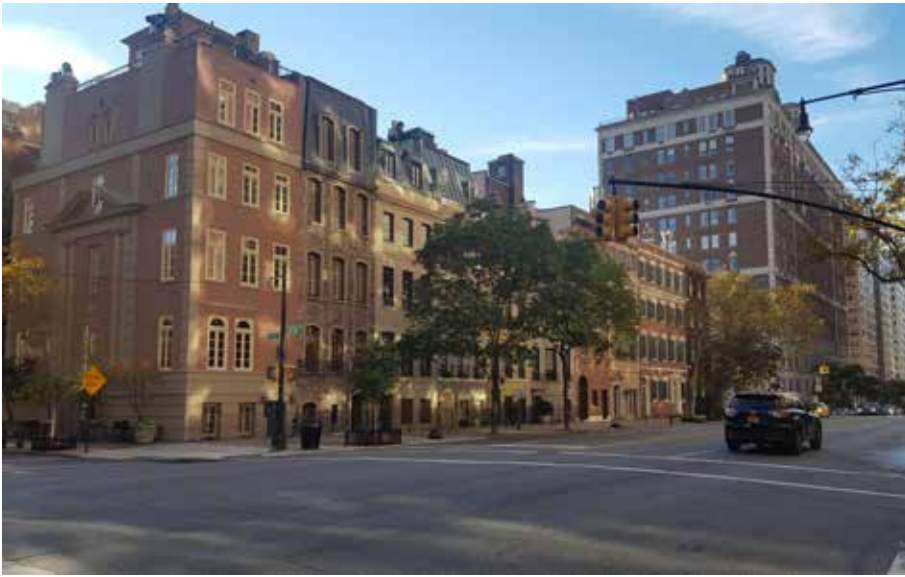
Photo 2.3-5 Sutton Place Historic District is developed mostly with 3-5 story buildings built to the street line
