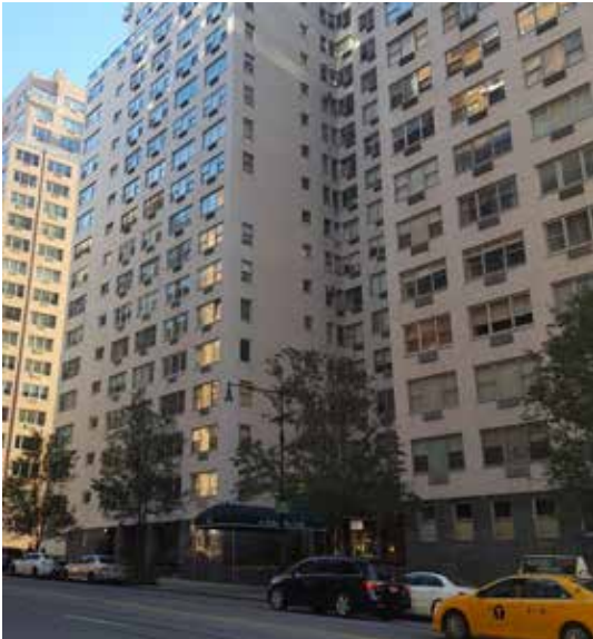
Photo 2.3-7 Cannon Point South (45 Sutton Place) has a recessed front courtyard
