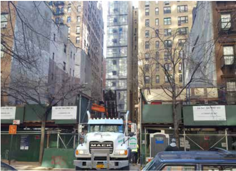
Photo 13 View of ongoing demolition at projected site 4a (photo captured February 6, 2017)
