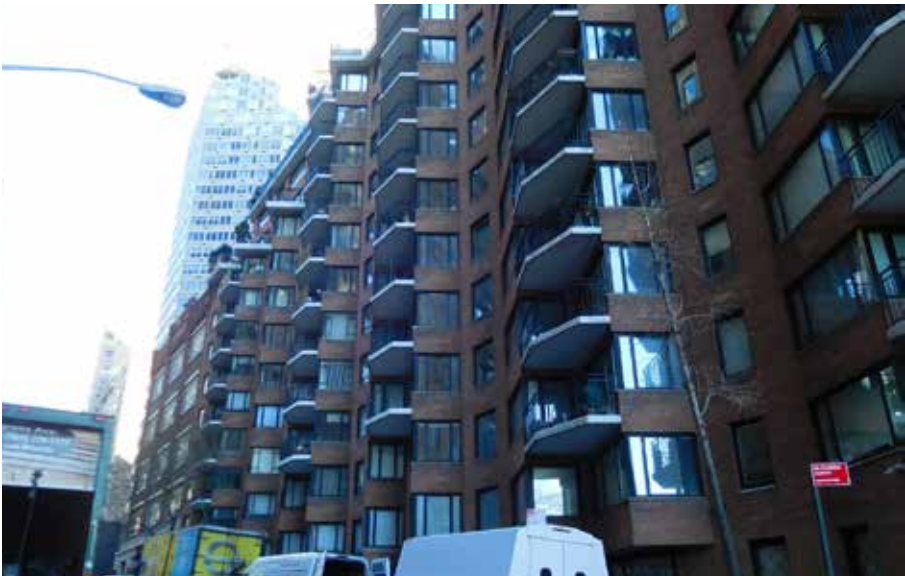
Photo 3 View of articulated facades on East 53rd between Sutton Place and 1st Avenue
