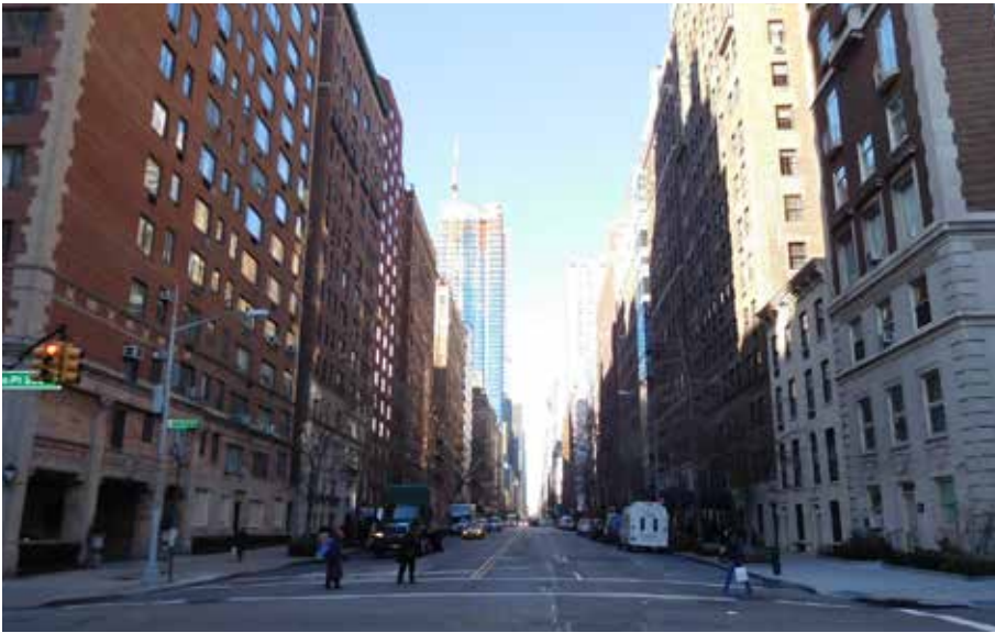
Photo 1 View of East 57th Street, Site 4c, and Site 1 looking west
