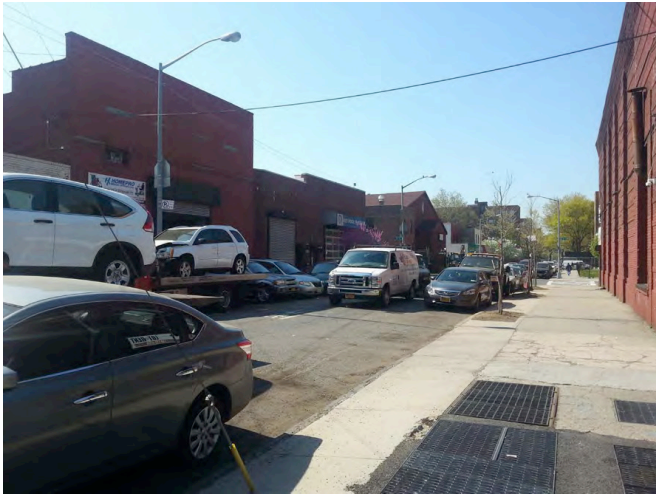
① VIEW FROM HICKS ST SOUTHWEST FACING BLOCK 535, JULY 1, 2015 NOT TO SCALE
