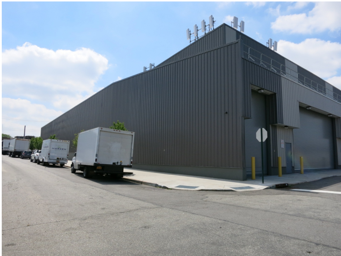
9. View of the intersection of 227th Street and 145th Road facing southeast.
