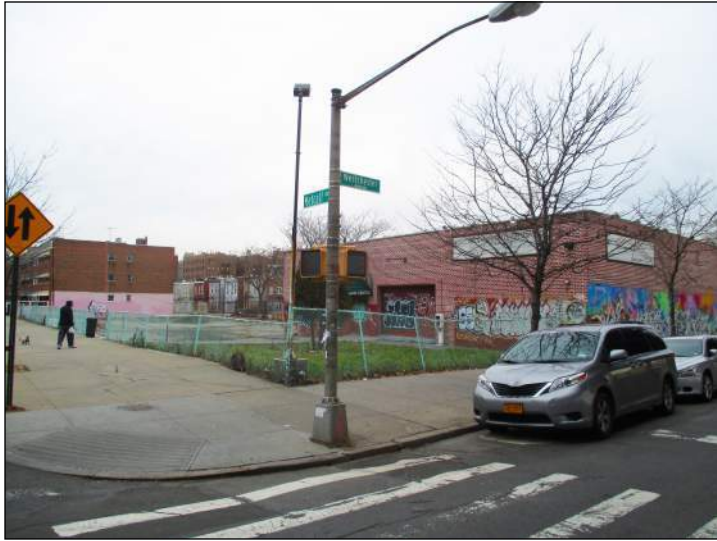
1. Projected development site 1, looking north-east from the corner of Westchester Avenue and Metcalf Avenue.
