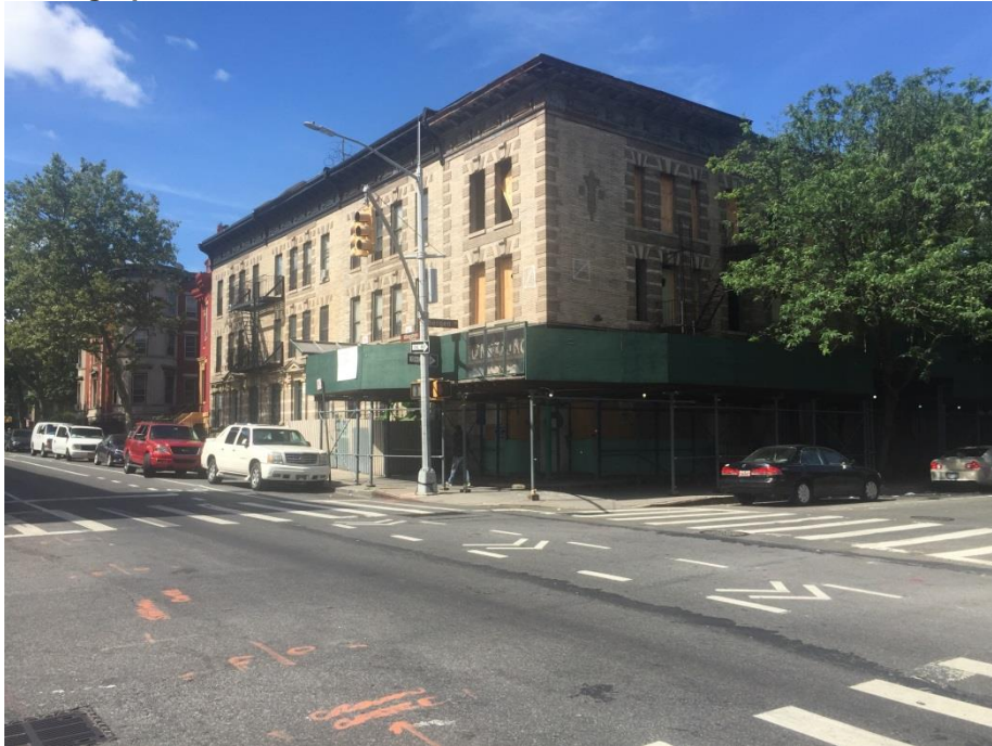
View of the Proposed Development Site at 120 Kingston Avenue
