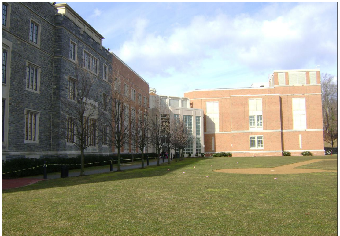
View west of Tillinghast Hall on the left and the Theater Building in the background 2
