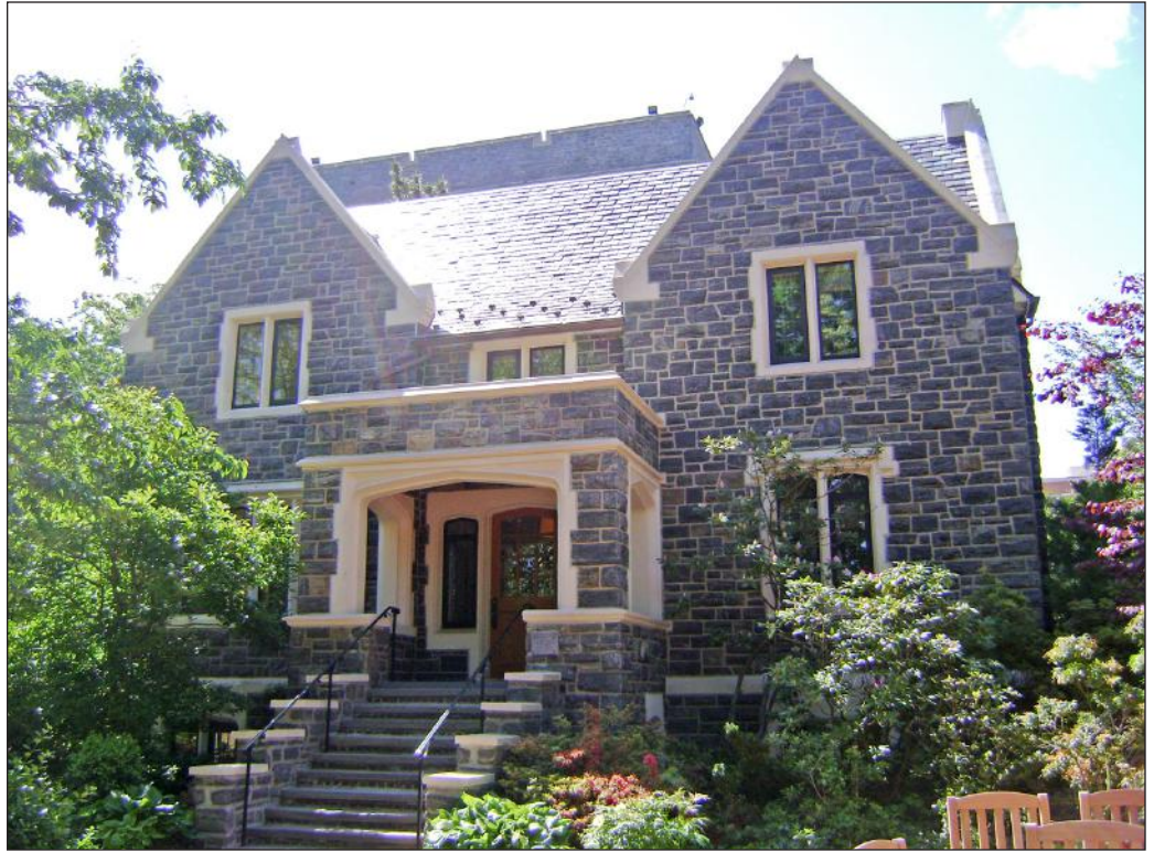
View of the front (east) elevation of Spence Cottage 9
