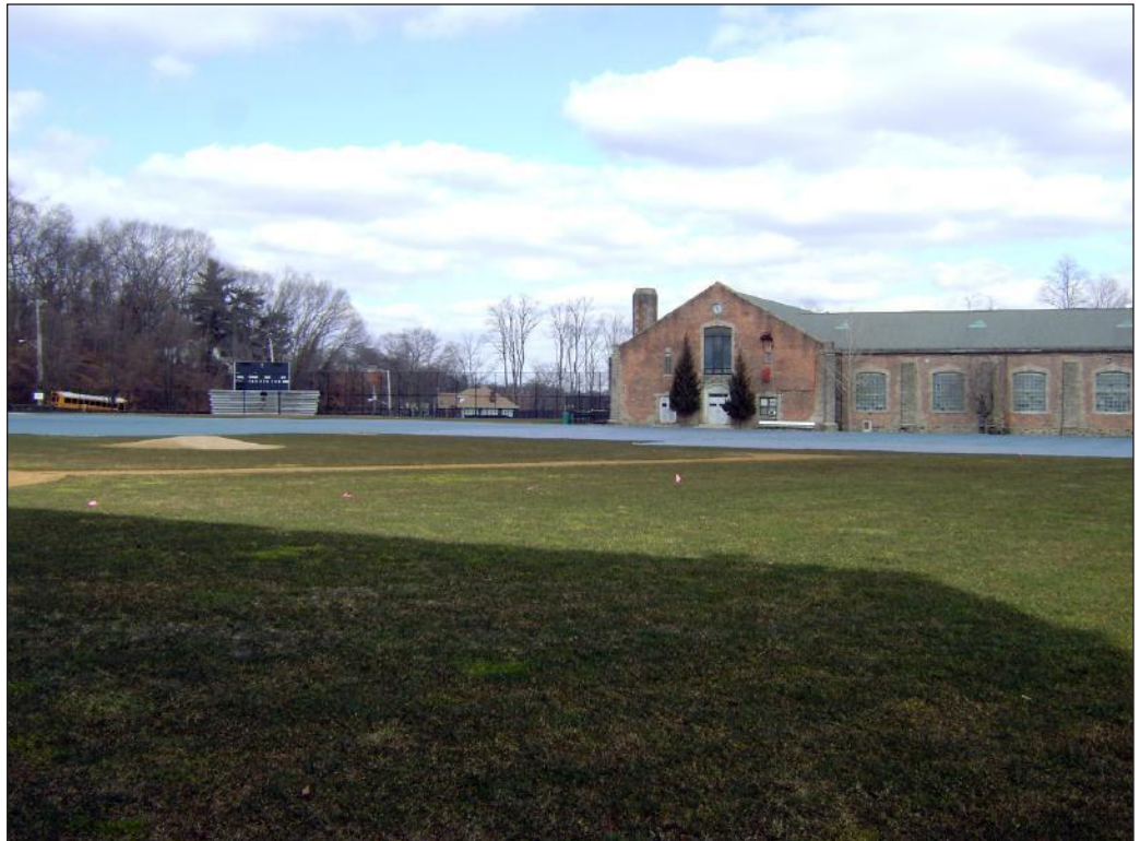
View of south façade of Prettyman Gym and playing field. The proposed Science Building would be located in the area left of the Gym 4
