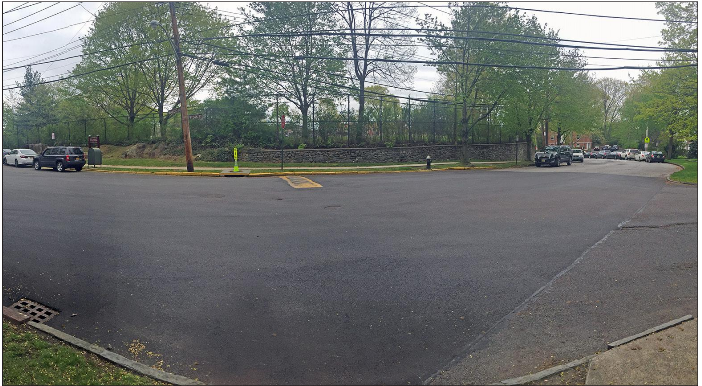
Four Acre Field as seen from West 246st Street, west of Waldo Avenue. 6 View looking northeast.
