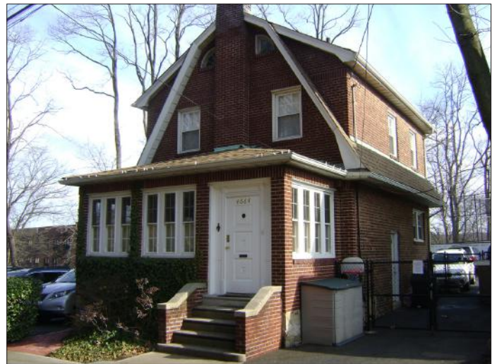
View northeast of one of the two houses on campus located at 4664 Tibbett Avenue 4b
