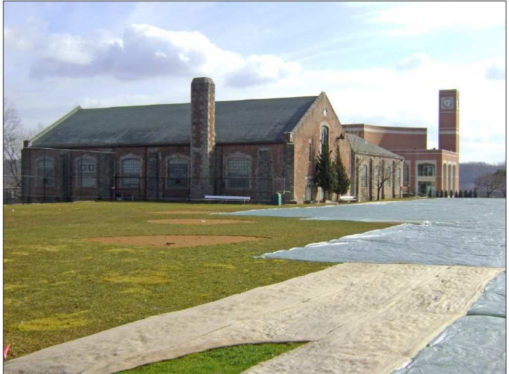
View east of Prettyman Gym and Fisher Hall 5
