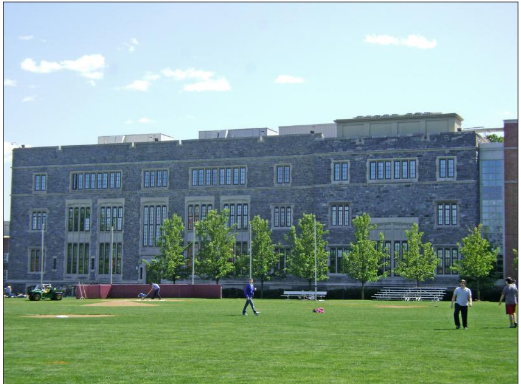
View of the north façade of Tillinghast Hall 6
