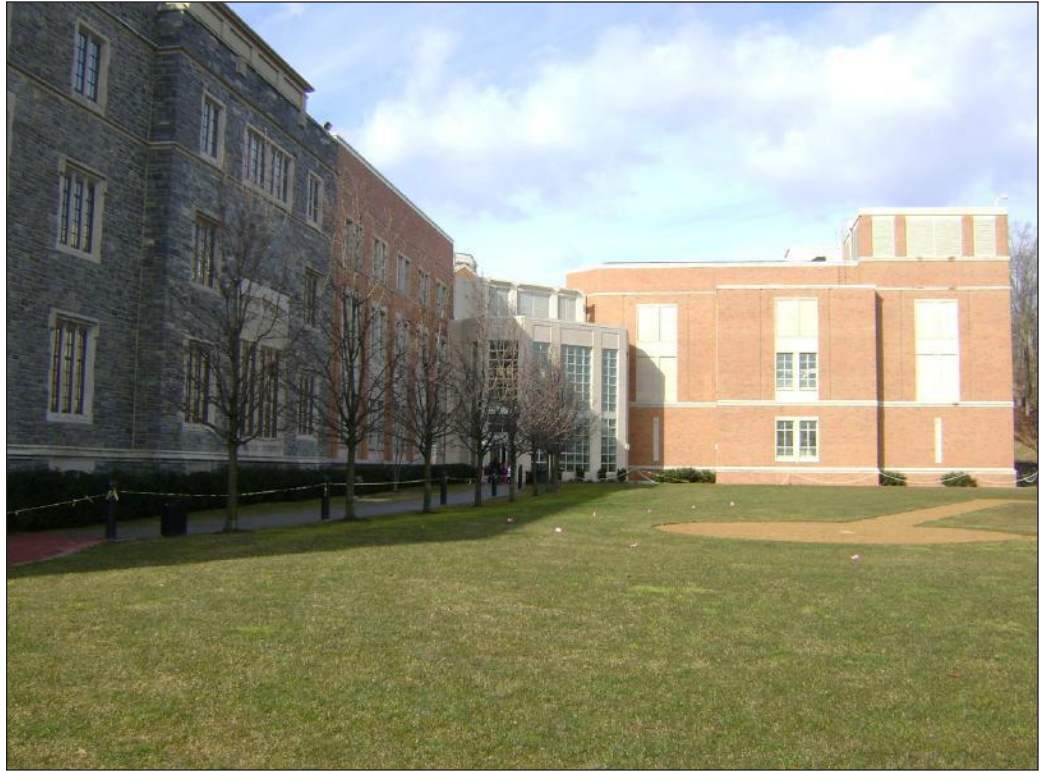
Oblique view west of the front facades of Tillinghast Hall and the Theater Building 1
