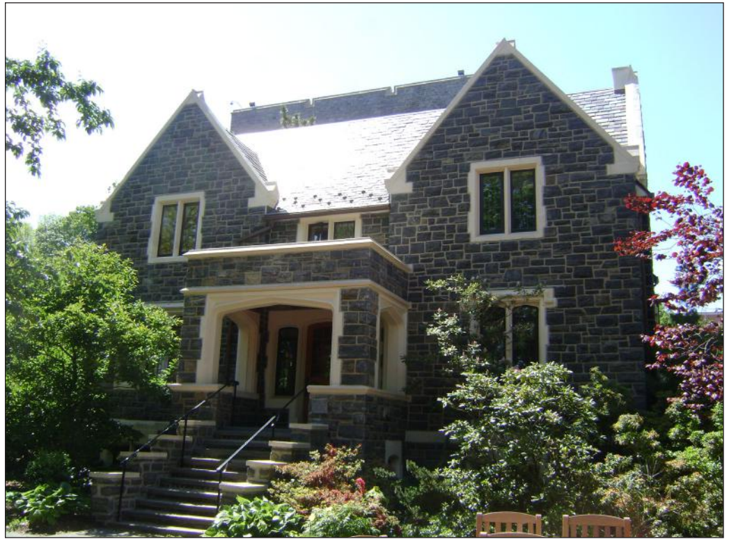
Spence Cottage located between Tillinghast and Pforzheimer Halls. View looking west. 5
