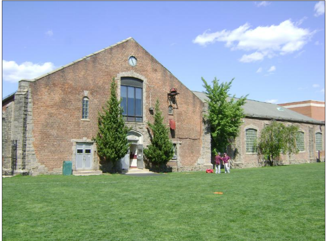
View of the south façade of Prettyman Gymnasium 5
