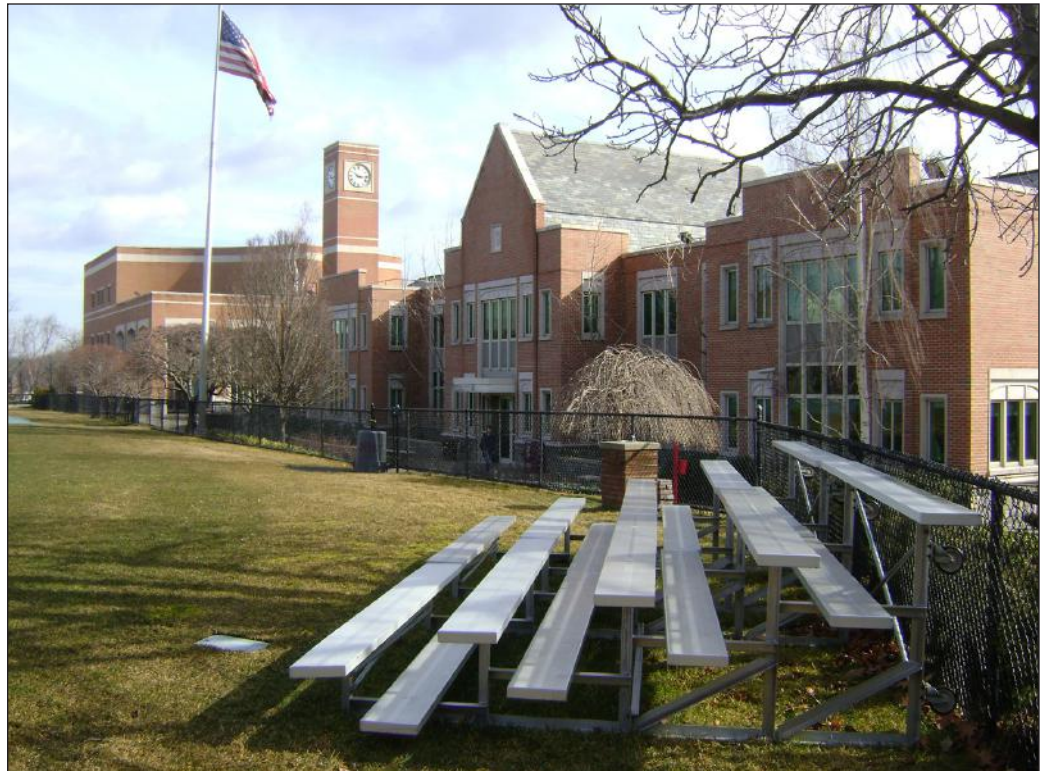
View northeast of Pforzheimer Hall in the foreground and Fisher Hall in the background 1
