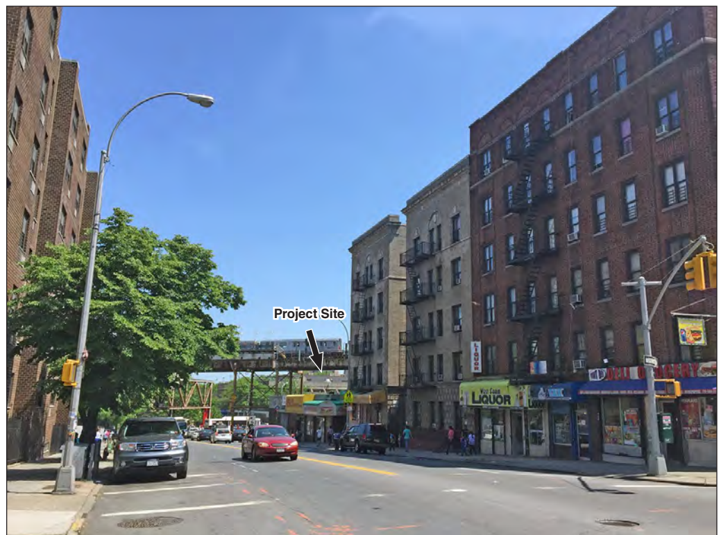
The one-story retail located on the project site as seen from East Tremont and Bryant Avenues, looking east. Two early 20th-century apartment buildings, located on the same block, are visible in the foreground with the elevated rail in the background 2
