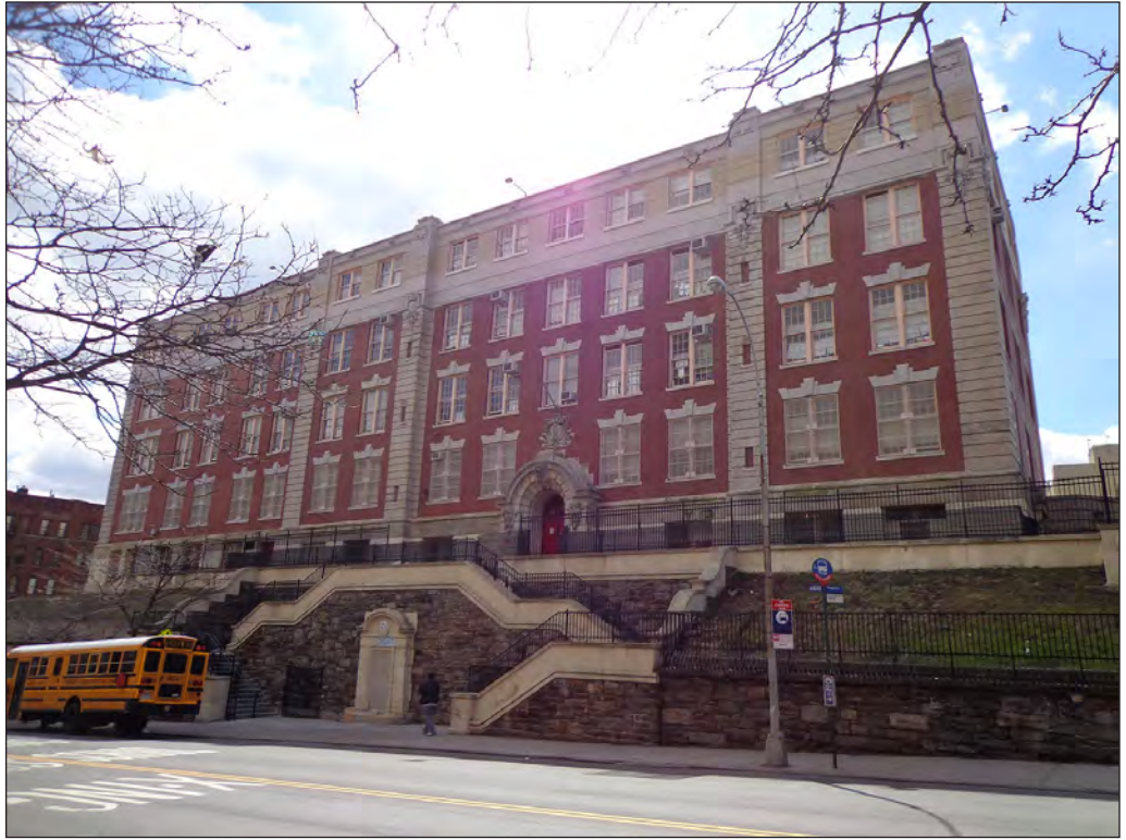
East Tremont Avenue façade 1
