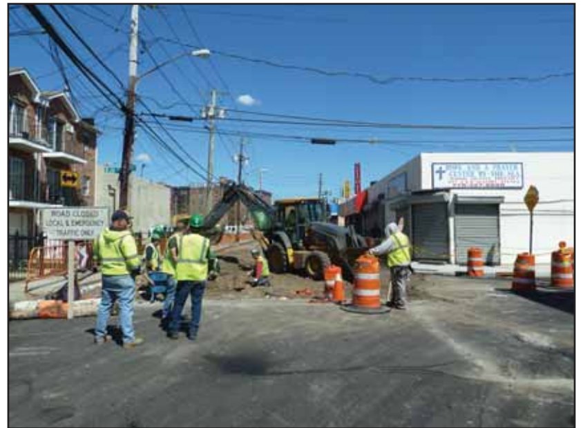
Construction on Seagirt Avenue (view east).
