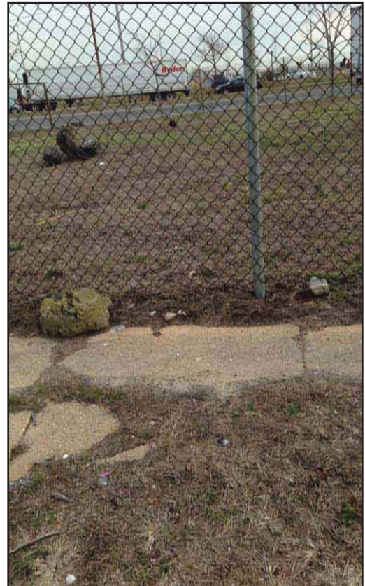
8. View south through Beach 13th St. site from Heyson Road.
