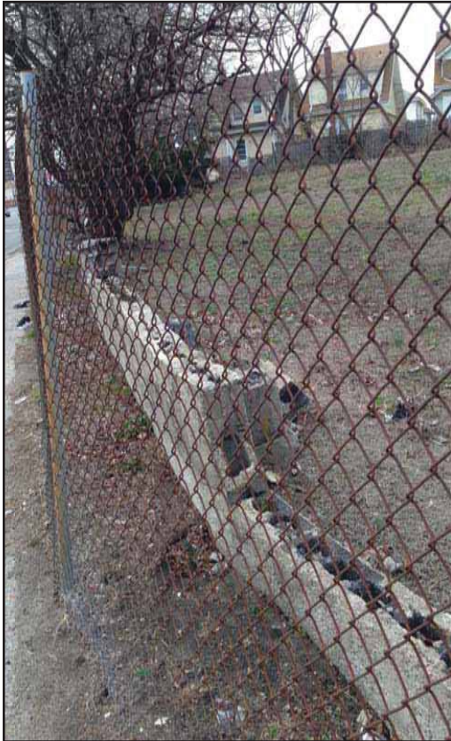
1. View northwest along Seagird Boulevard through Fernside Pl. site. Residences along Highland Court visible in background.
