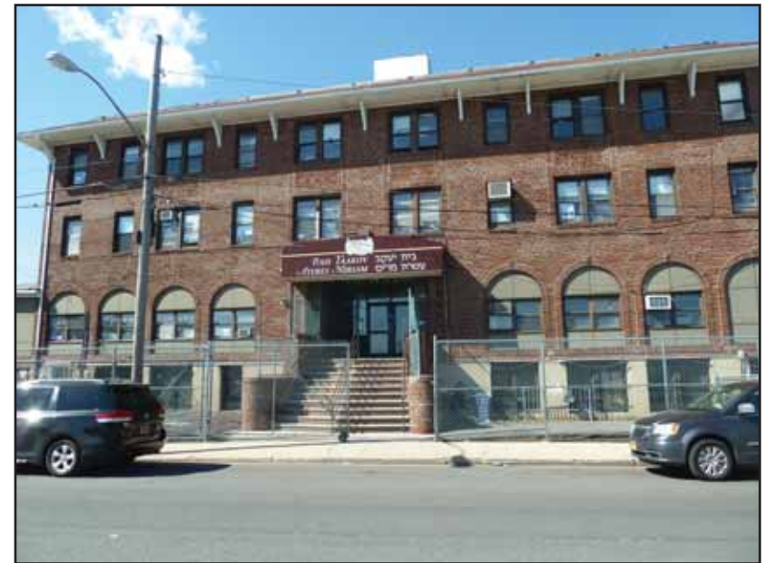
Bais Yaakov Ateres Miriam private school at the northeast corner of Beach 13th Street and Heyson Road.
