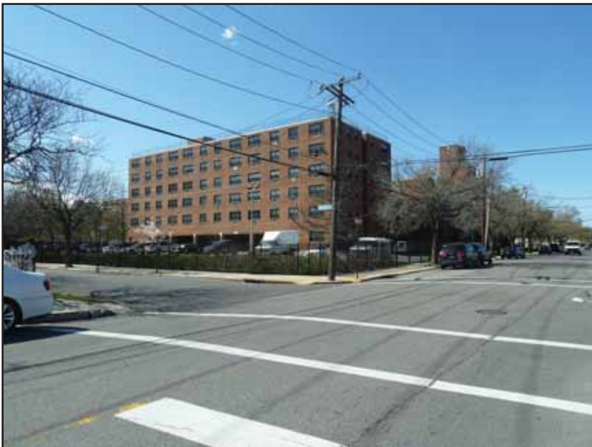
Multi-family residential development on the northwest corner of Beach 13th Street and Heyson Road.
