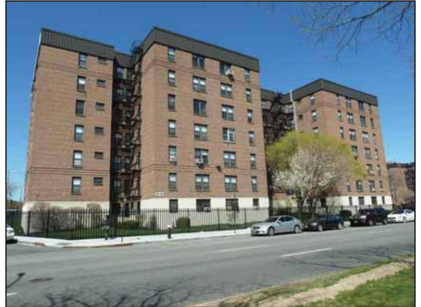
Multi-family residential development on the east side of Fernside Place.
