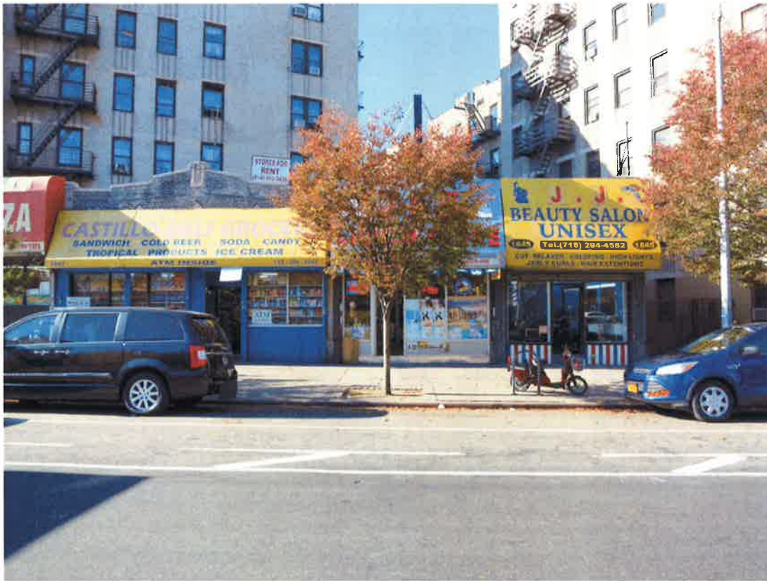
3. 1845 Grand Concourse - Existing conditions - daylight. (2 of 2)
