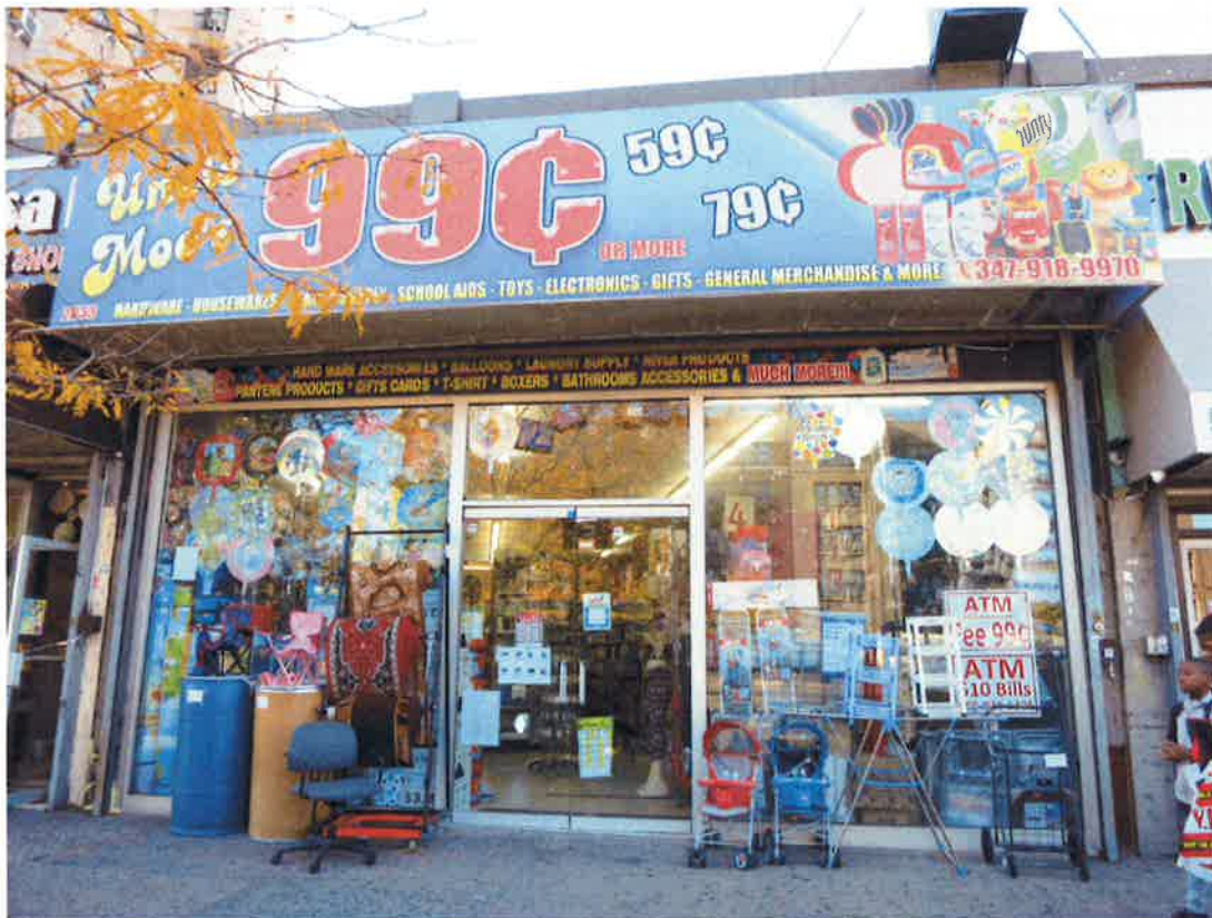
6. 2029-2043 Grand Concourse - Existing conditions - daylight. (4 of 6)
