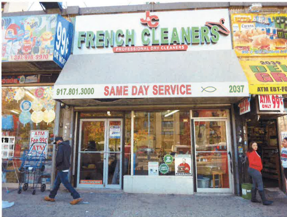
6. 2029-2043 Grand Concourse - Existing conditions - daylight. (3 of 6)
