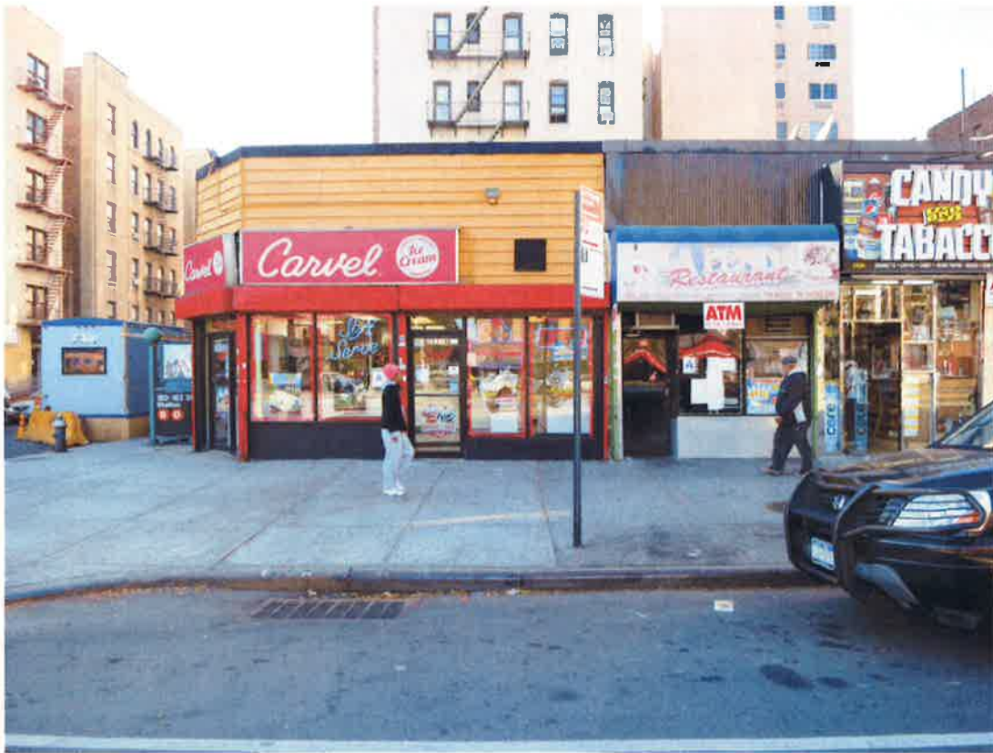
9, 2231-2233 Grand Concourse - Existing conditions - daylight.
