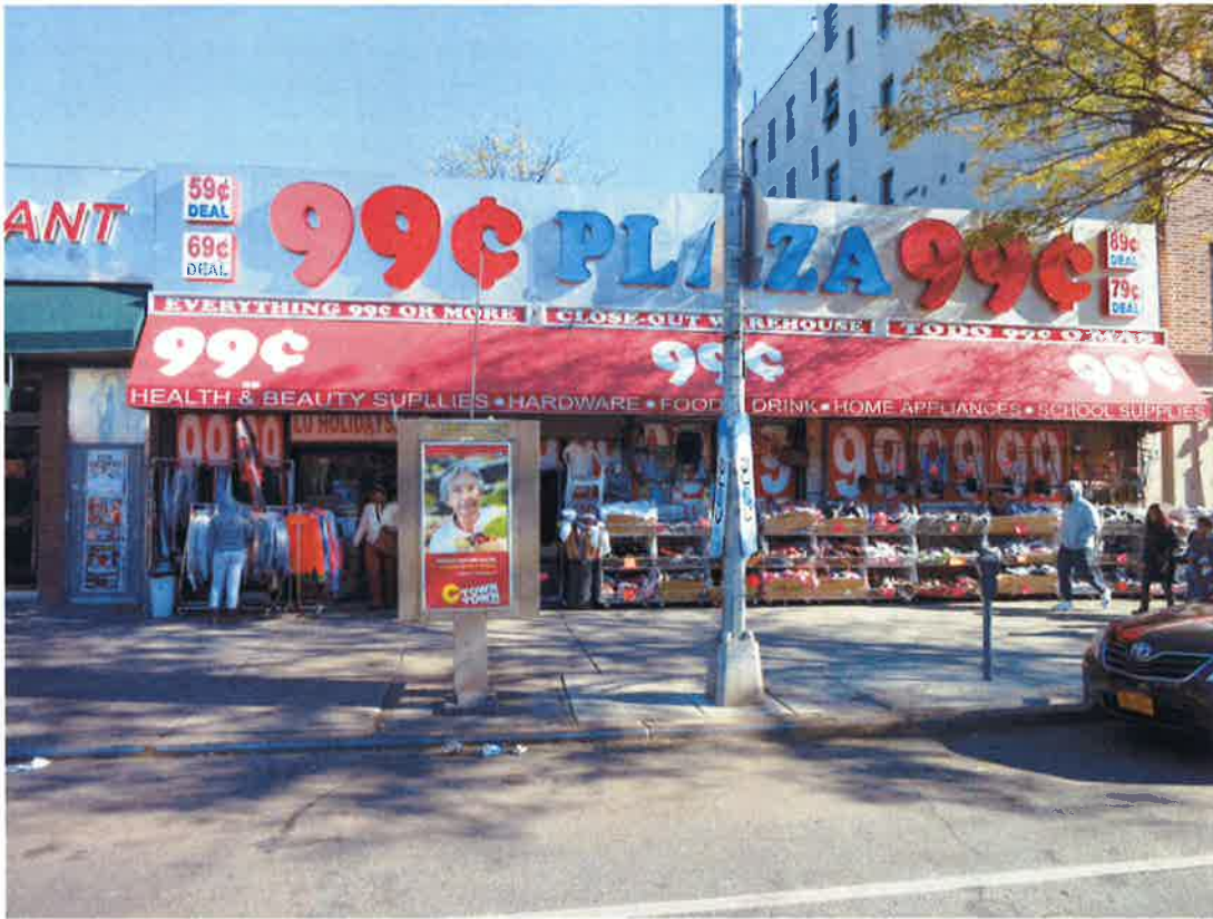
11. 2262-2268 Grand Concourse - Existing conditions - daylight. (1 of 4)
