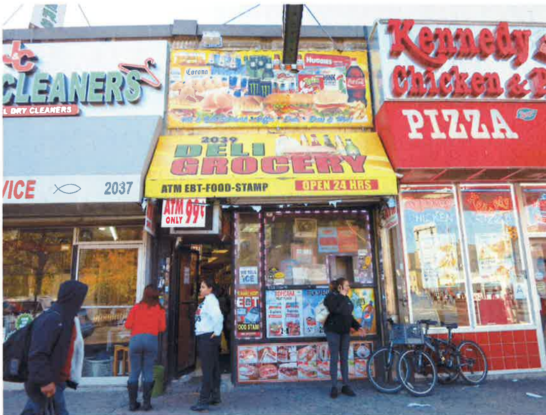
6. 2029-2043 Grand Concourse - Existing conditions - daylight. (2 of 6)
