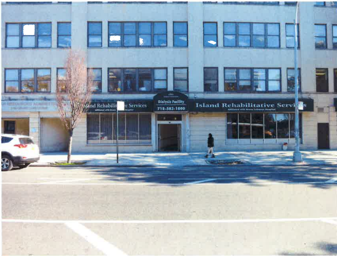
2. 1780 Grand Concourse - Existing conditions - daylight. (1 of 2)
