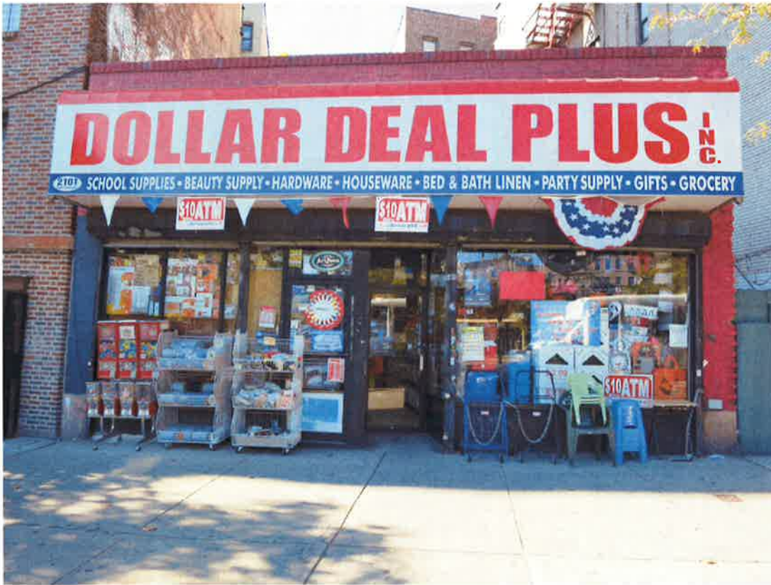
7. 2101 Grand Concourse - Existing conditions - daylight.
