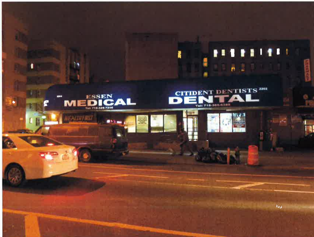
8. 2202 Grand Concourse - Existing conditions - after dark.
