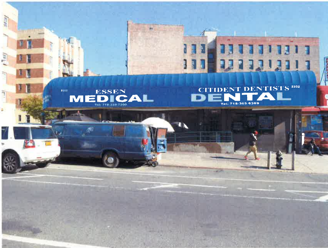
8. 2202 Grand Concourse - Existing conditions - daylight.
