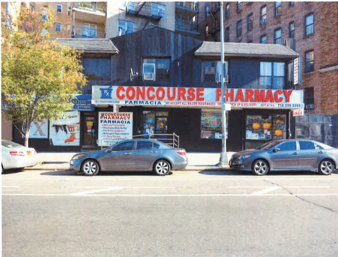
4. 1850 Grand Concourse - Existing conditions - daylight.
