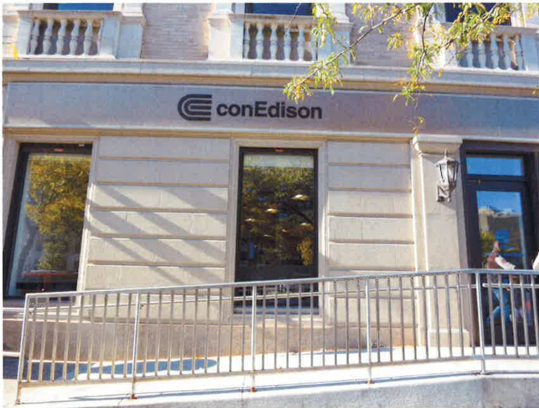
1. 1775 Grand Concourse - Existing conditions - daylight. (1 of 4)
