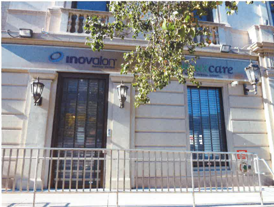
1. 1775 Grand Concourse - Existing conditions - daylight. (3 of 4)
