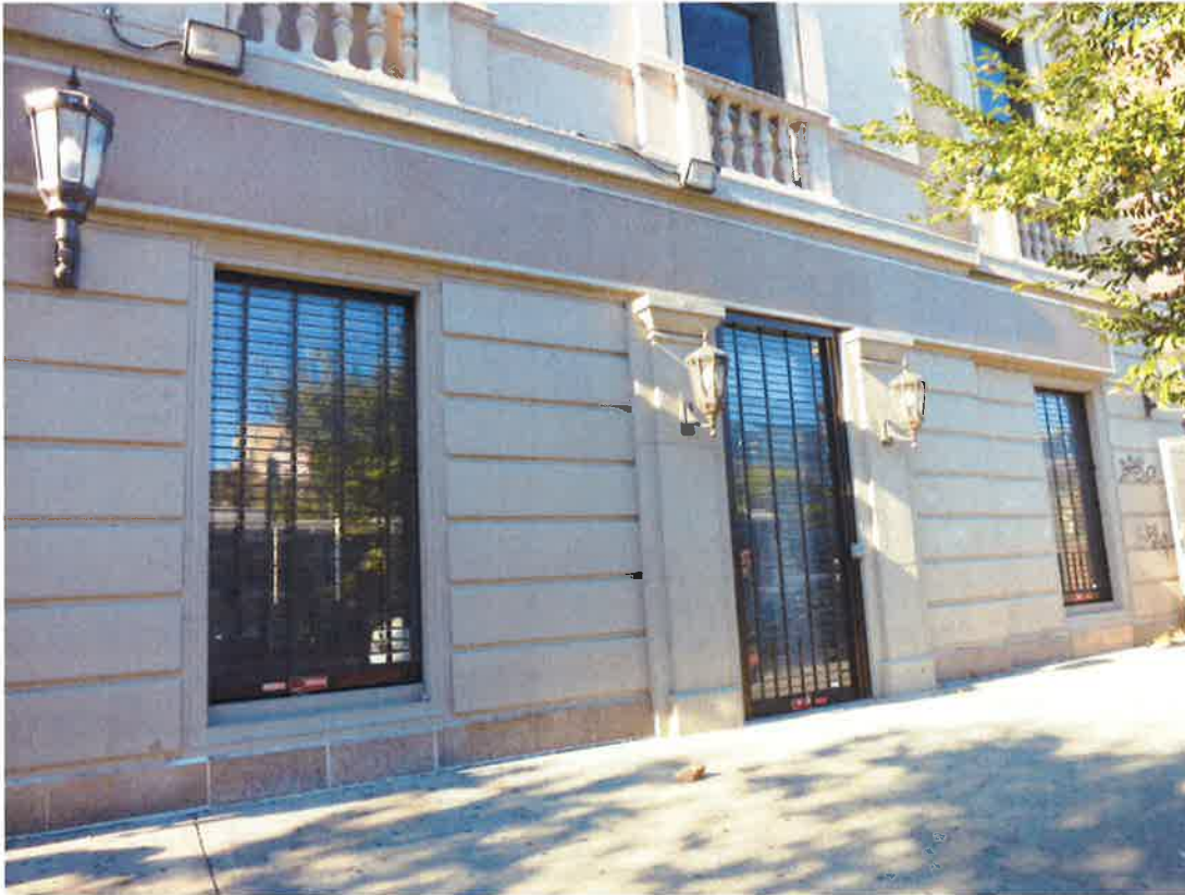
1. 1775 Grand Concourse - Existing conditions - daylight. (4 of 4)
