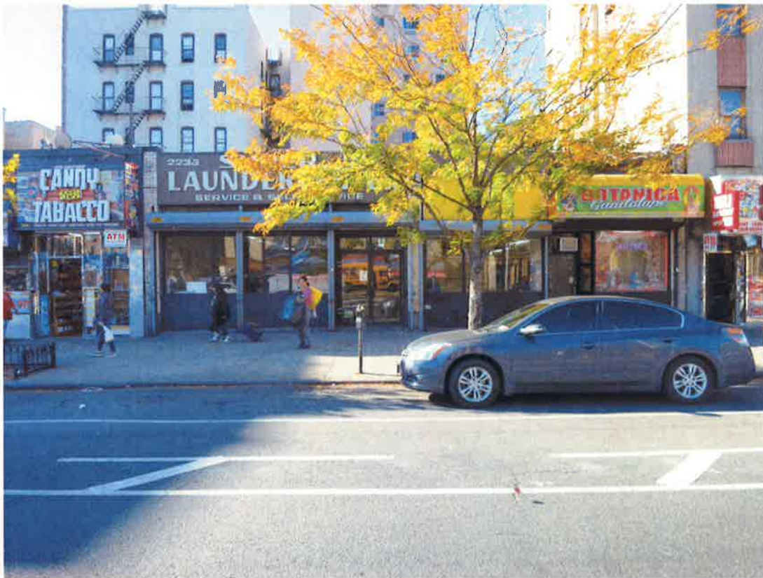
10. 2235-2237 Grand Concourse - Existing conditions - daylight.
