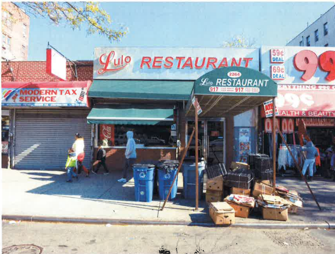
11. 2262-2268 Grand Concourse - Existing conditions - daylight. (2 of 4)
