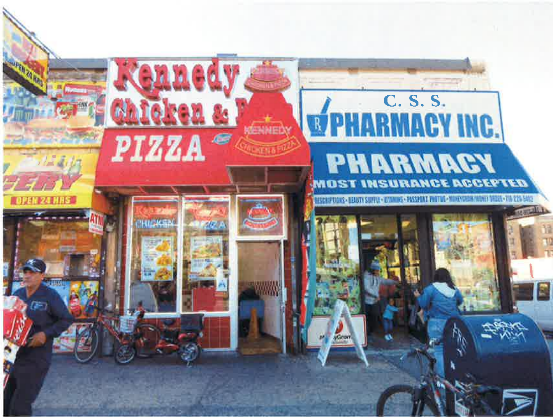
6. 2029-2043 Grand Concourse - Existing conditions - daylight. (1 of 6)
