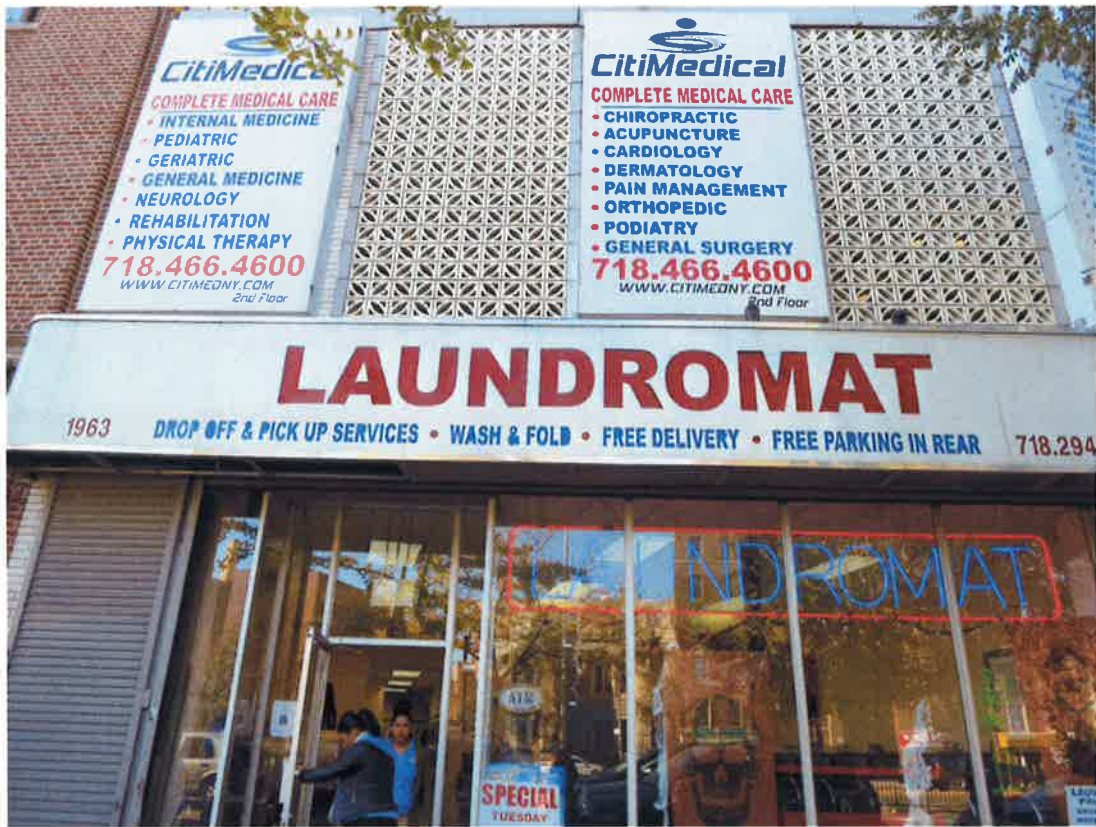
5. 1963 Grand Concourse - Existing conditions - daylight. (3 of 3)
