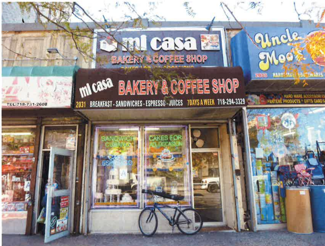
6. 2029-2043 Grand Concourse - Existing conditions - daylight. (5 of 6)
