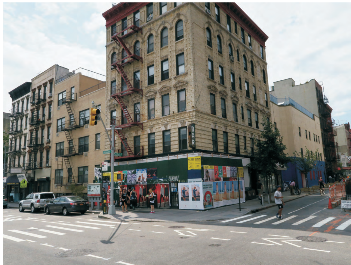
15. View of the intersection of East Houston Street and Suffolk Street facing southeast.
