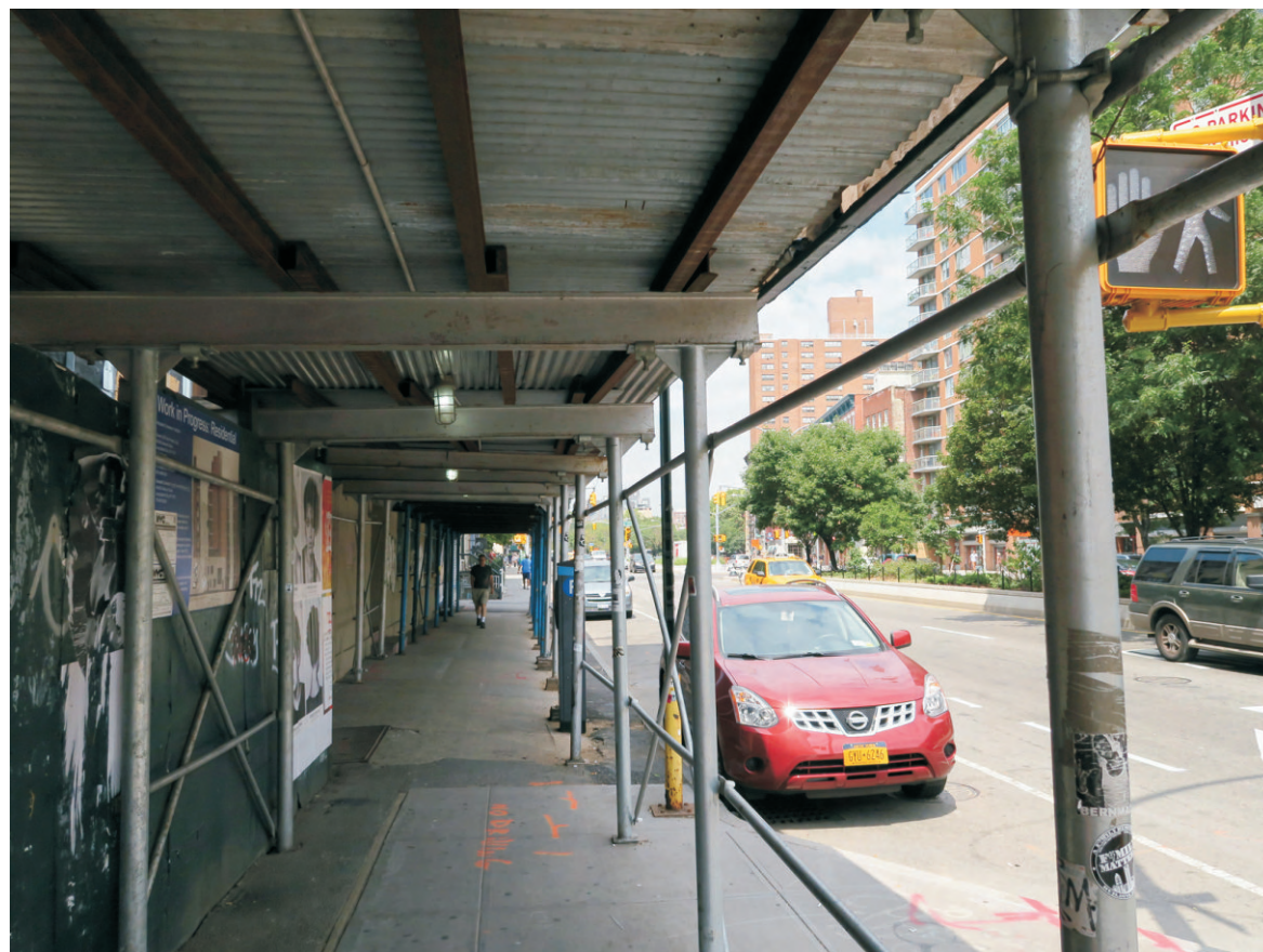
12. View of the sidewalk along the south side of East Houston Street facing west from Suffolk Street (Site at left).
