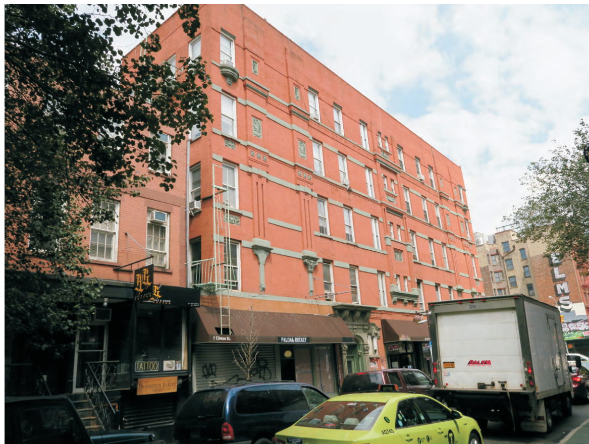
27. View of the side of Clinton Street facing northwest.
