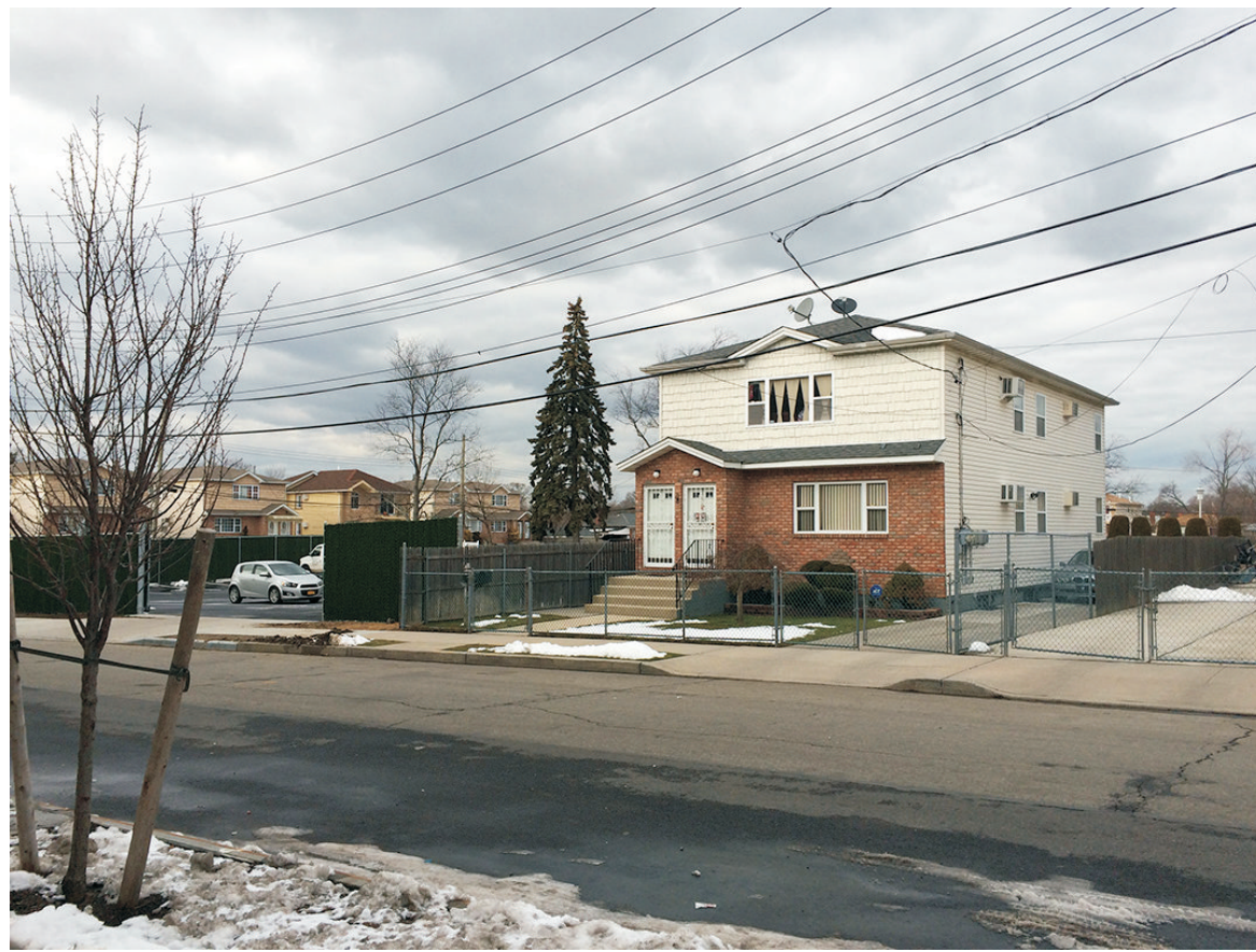
1. View of the Site facing northwest from 145th Road.
