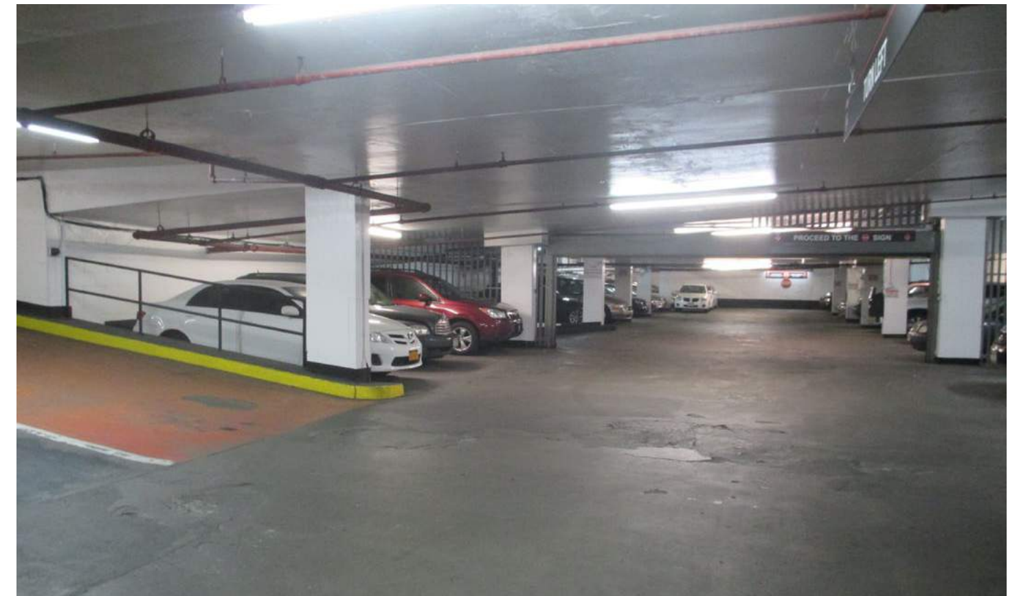
3. Existing conditions inside Knickerbocker Plaza parking garage. April 29, 2016.
