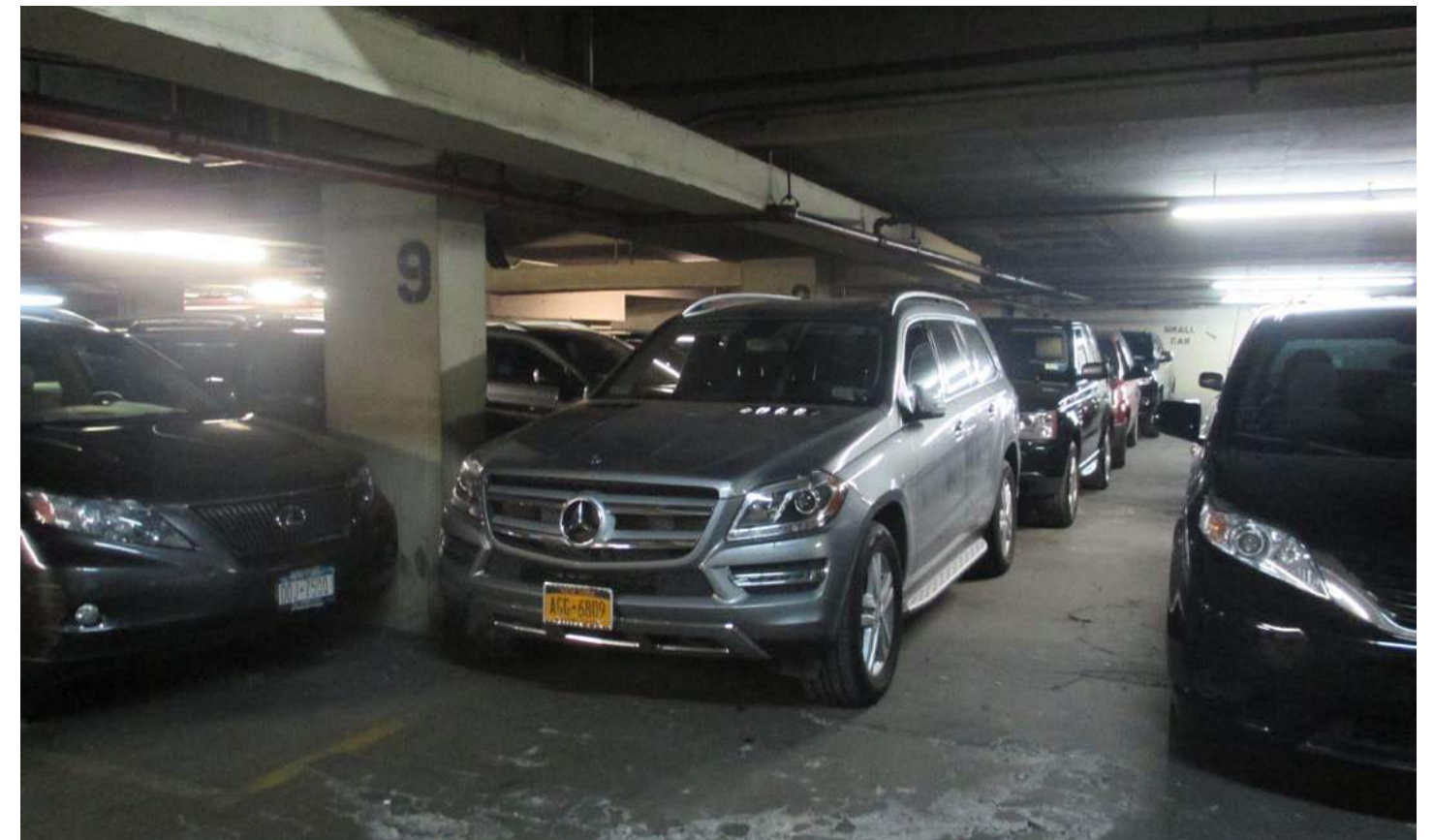
3. Existing conditions inside Yorkville Tower parking garage. April 29, 2016.
