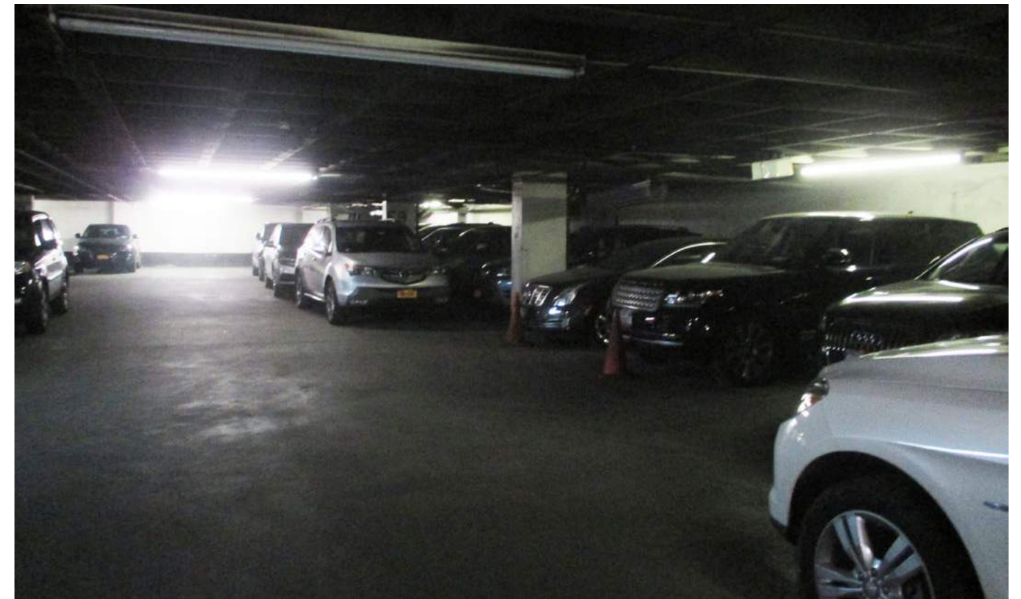
3. Existing conditions inside Ruppert Tower parking garage. April 29, 2016.
