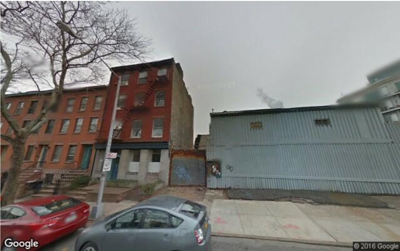
75-77 Gold Street, Area II, Vinegar Hill Historic District
