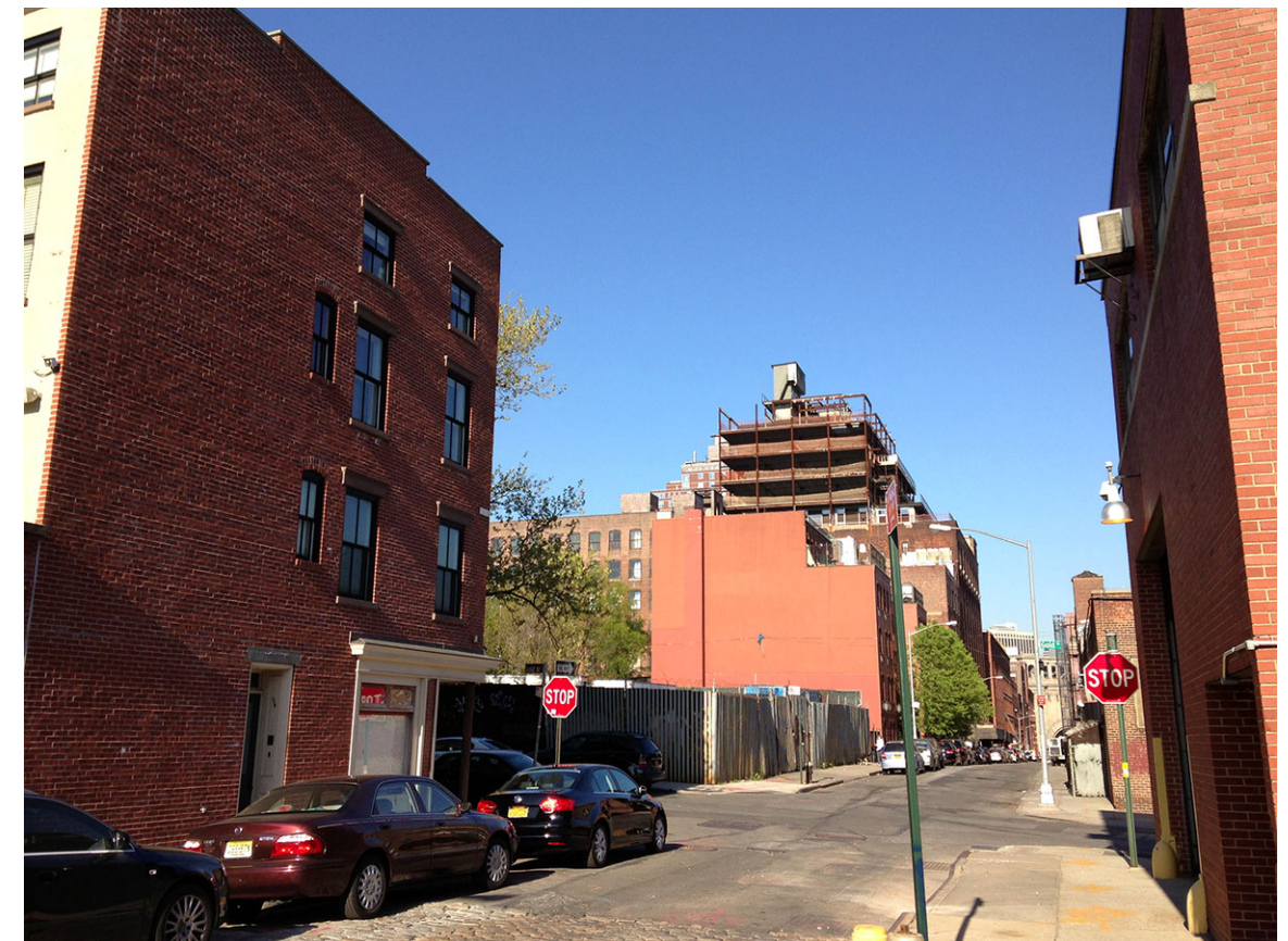
4. LOOKING WEST FROM WATER STREET
