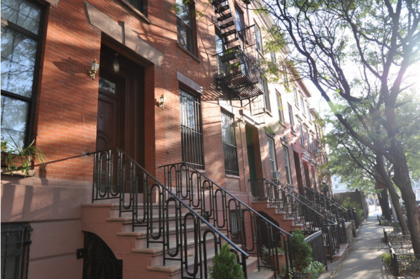
Front Street, Area I, Vinegar Hill Historic District
