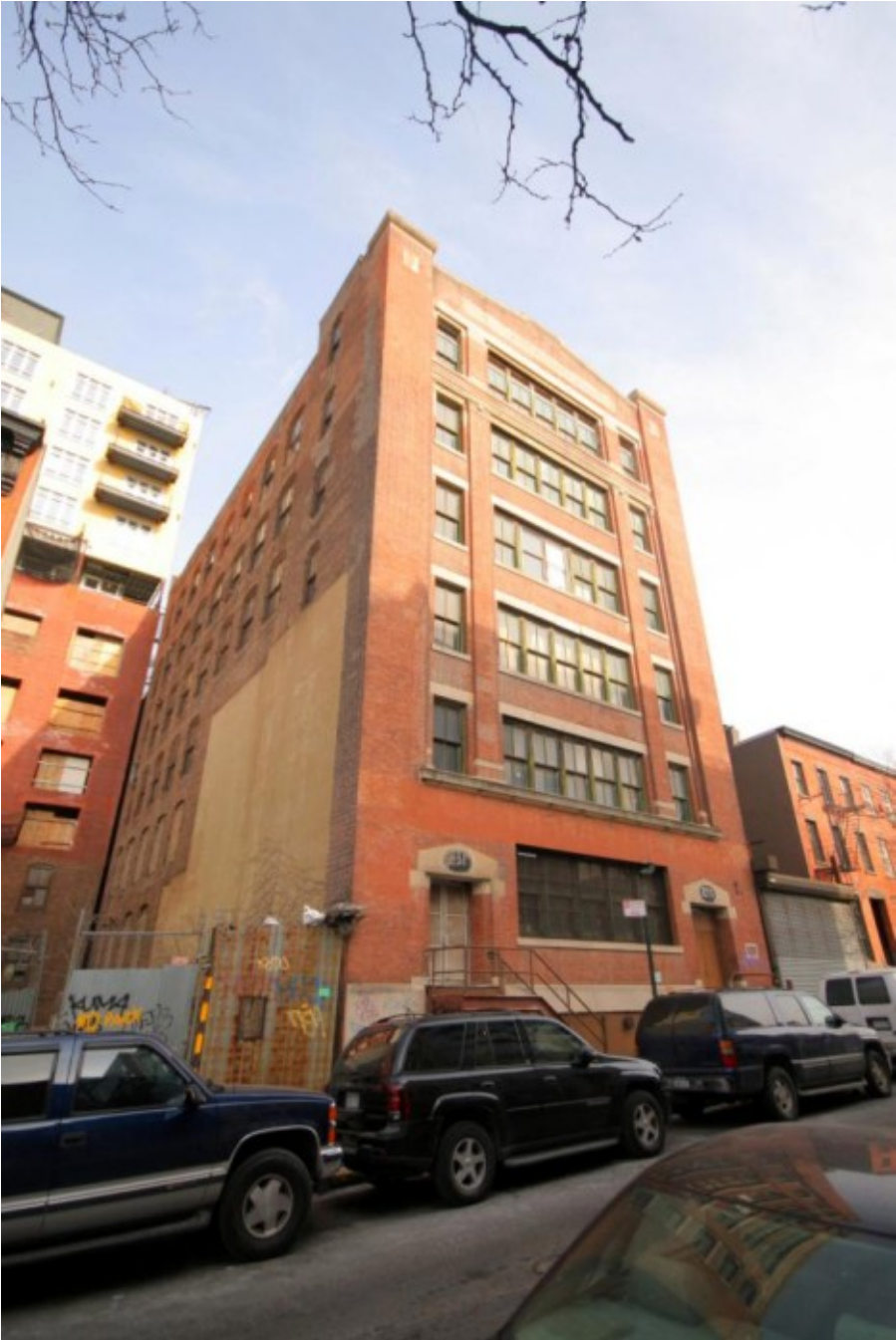
231-233 Front Street, Area I, Vinegar Hill Historic District
