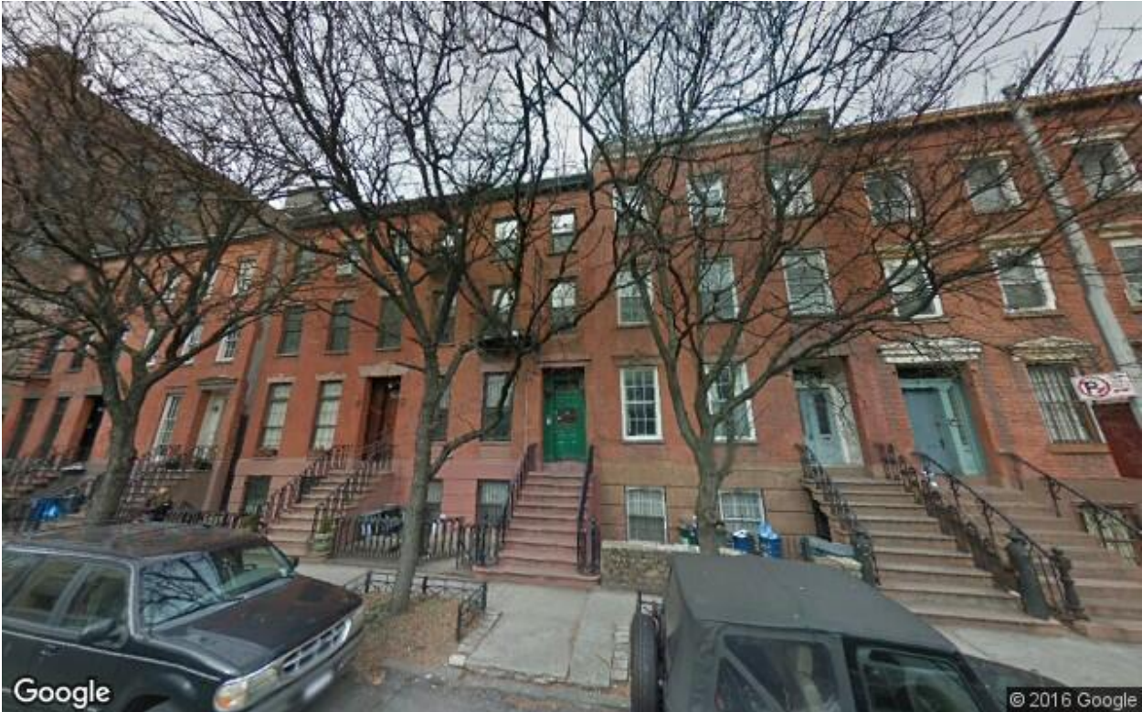
Front Street, Area I, Vinegar Hill Historic District
