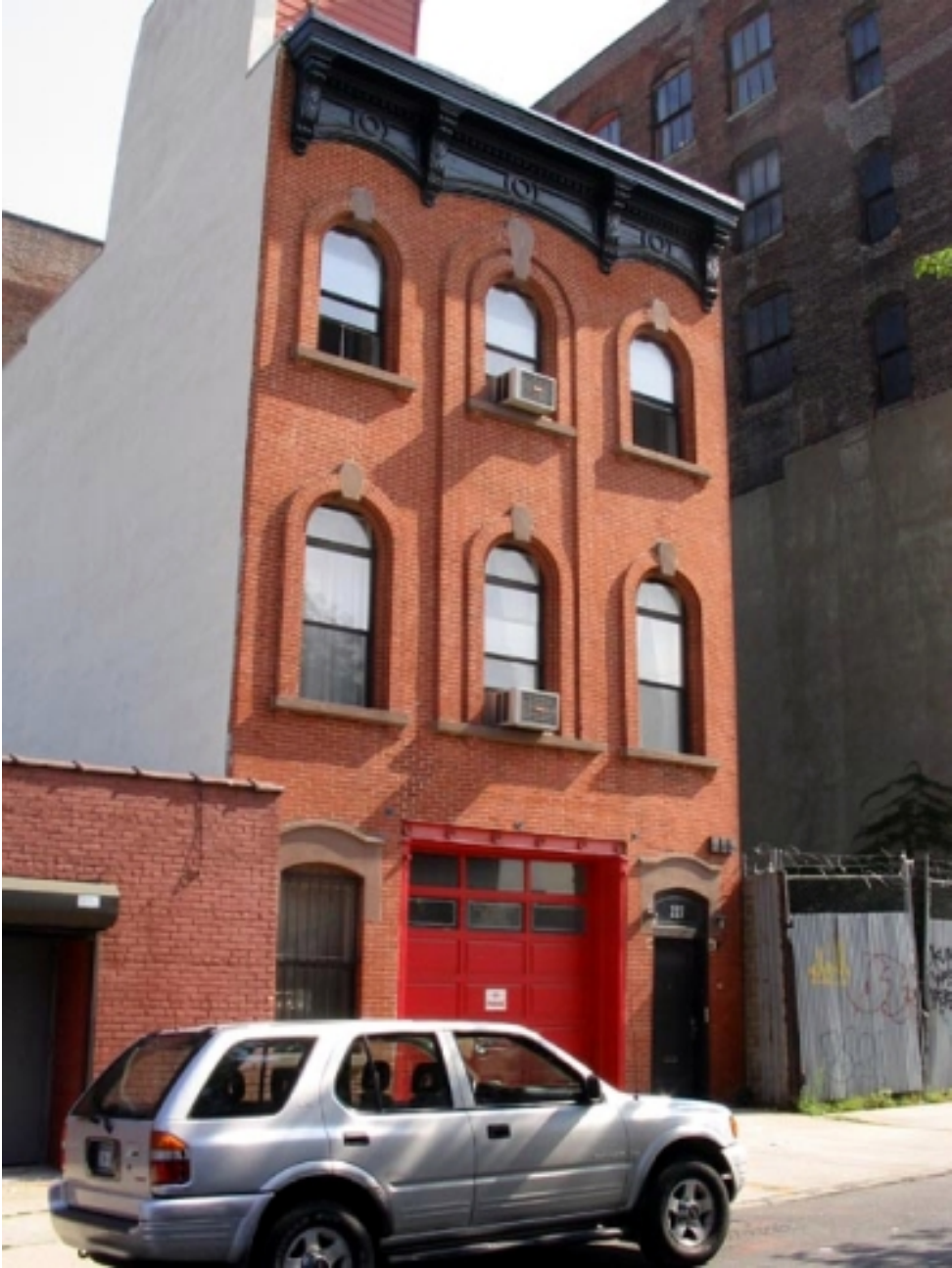
227 Front Street, Area I, Vinegar Hill Historic District
