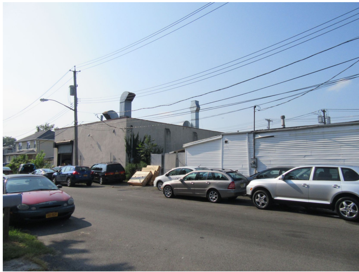
4. View of the Development Site facing northwest from Clifton Street.
