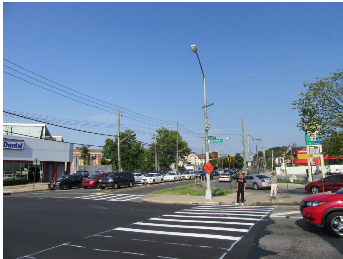
12. View of Victory Boulevard facing east from Richmond Avenue.
