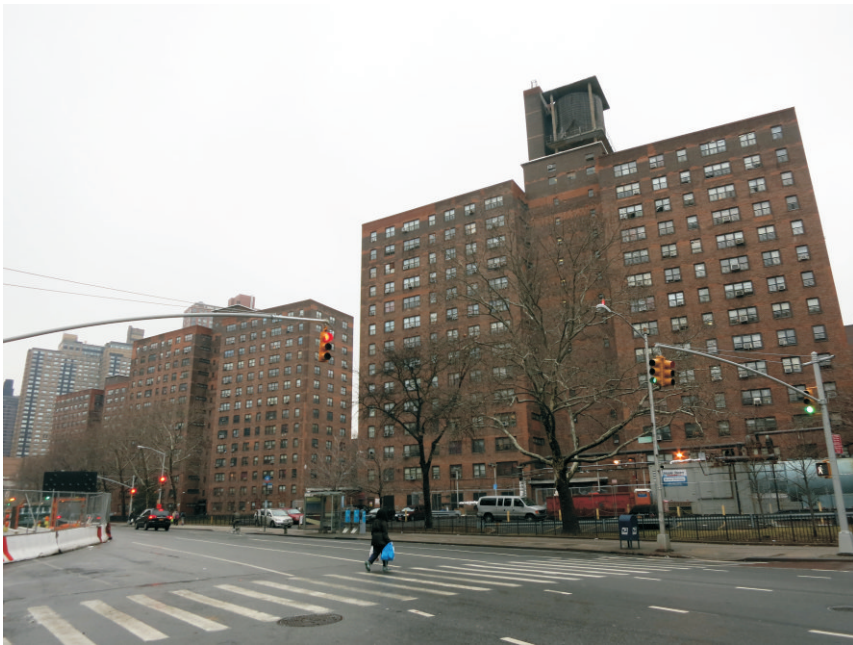
16. View of the west side of Second Avenue between East 100th Street and East 101st Street.
