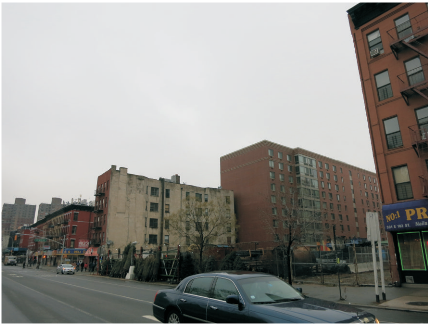
1. View of the east side of Second Avenue between East 102nd Street and East 103rd Street.
