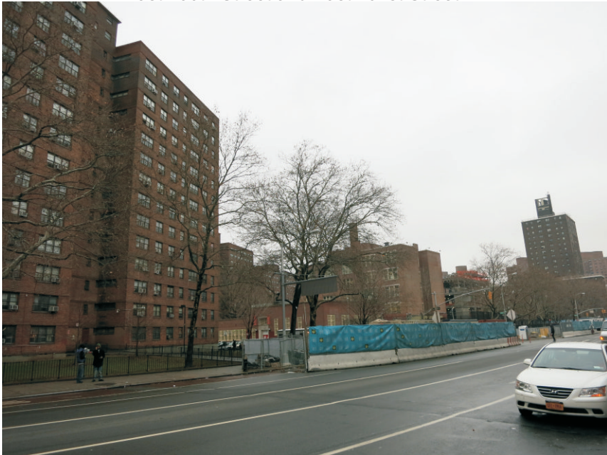
18. View of the west side of Second Avenue between East 101st Street and East 102nd Street.
