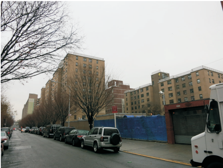
6. View of the south side of East 102nd Street between First Avenue and Second Avenue.
