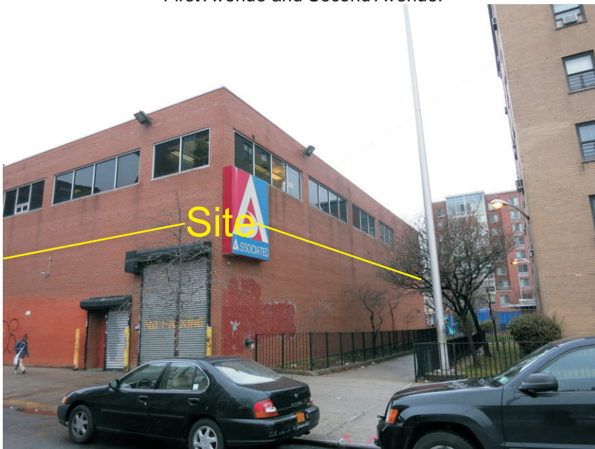
15. View of the north side of East 101st Street between First Avenue and Second Avenue.
