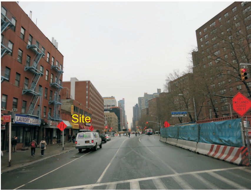
7. View of Second Avenue facing south from East 102nd Street.
