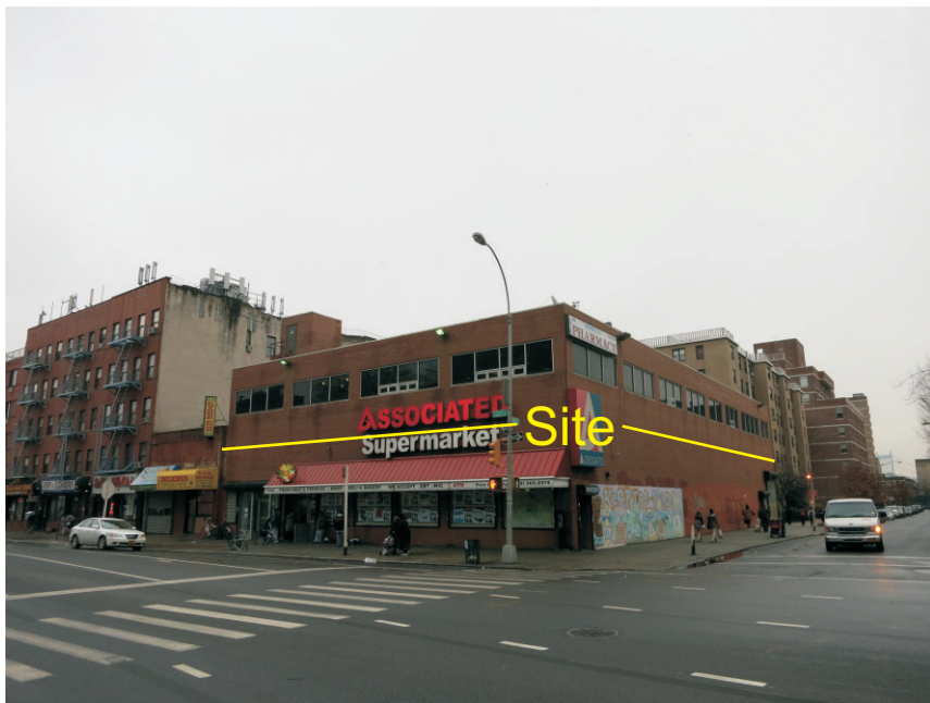
10. View of the northeast corner of Second Avenue and East 101st Street.
