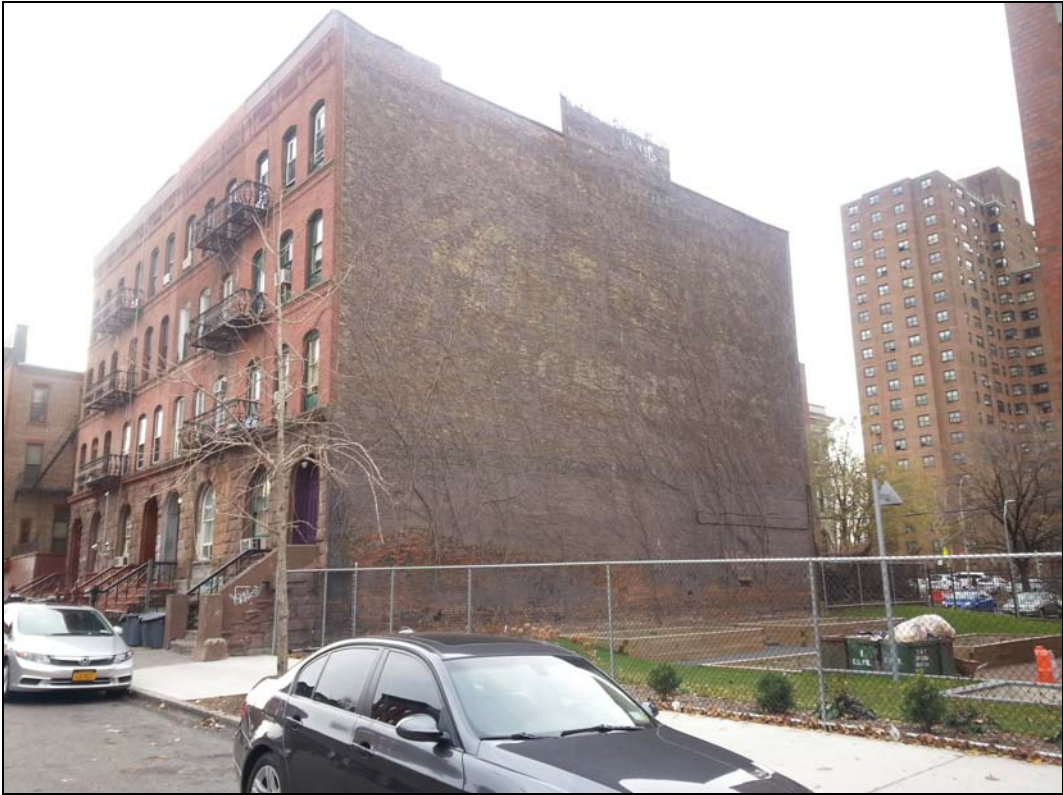
Western party wall of 302 East 139 th Street adjacent to Project Site
