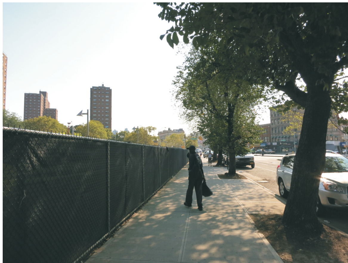
18. View of the sidewalk along the southeast side of 3rd Avenue facing southwest (Site at left).
