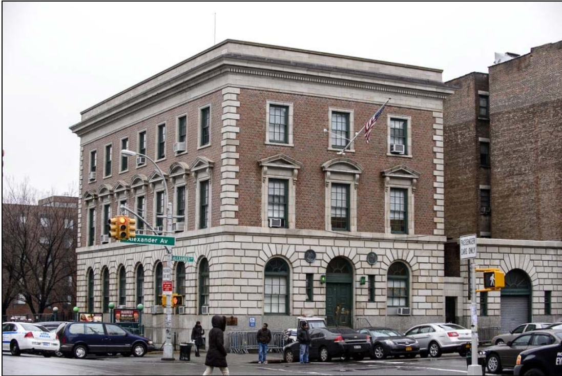
40 th Precinct from southeast. Project site is visible at left.
