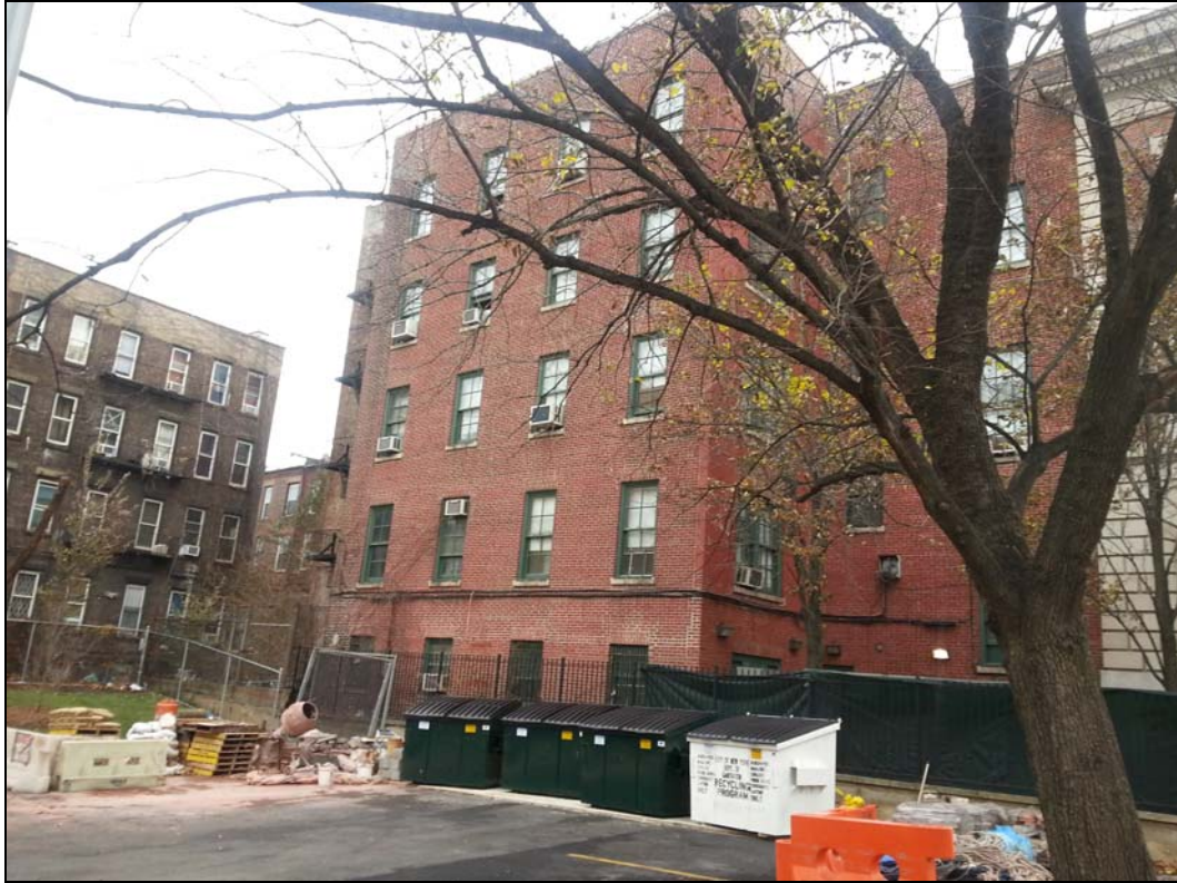
Western façade of Police Station from Project Site
