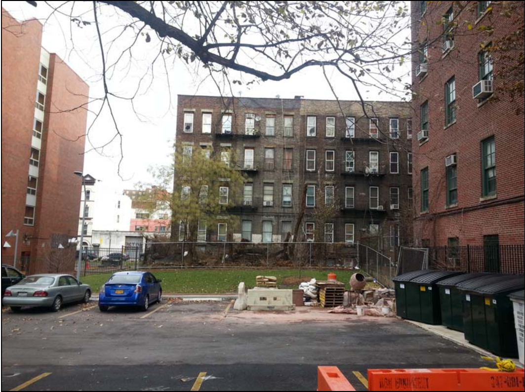
Rear of 302-308 East 139 th Street from Project Site. Western Façade of Police Station is at right.
