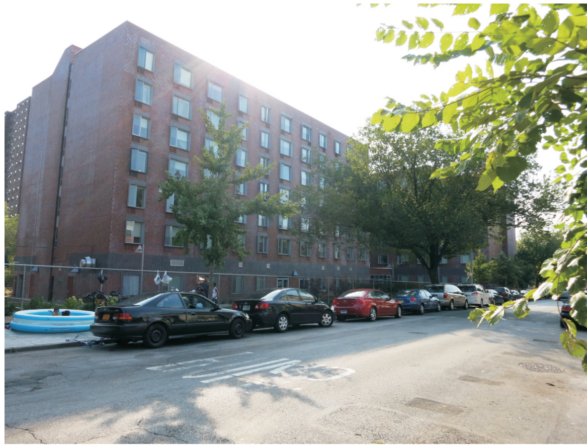
25. View of the Site facing west from East 139th Street.
