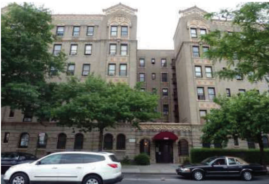
3 Existing mixed-use building on Risse Street (Lot 22).
