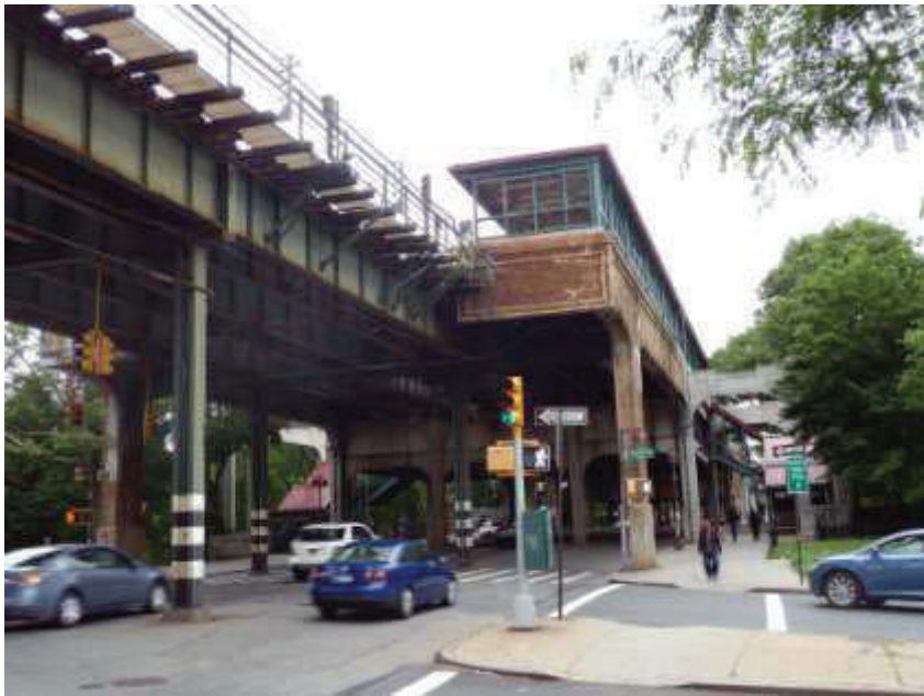
5 Elevated IRT Subway Tracks over Jerome Avenue.
