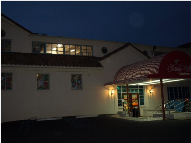
PARKING LOT AWNING CLOSE-UP
