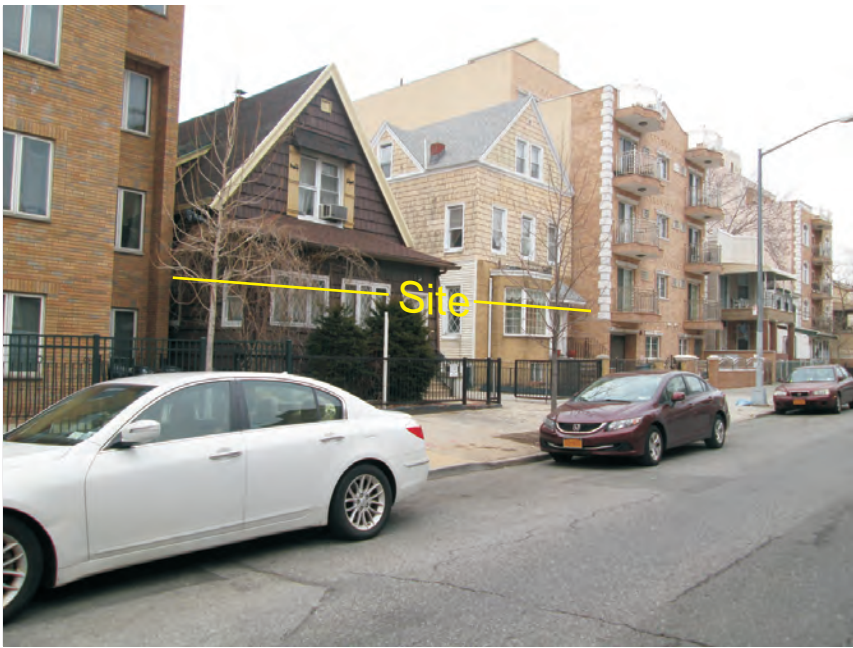
4. View of the Site from 38th Street, facing northwest.
