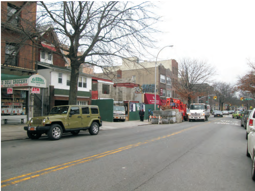
12. View of 31st Avenue, facing southwest.
