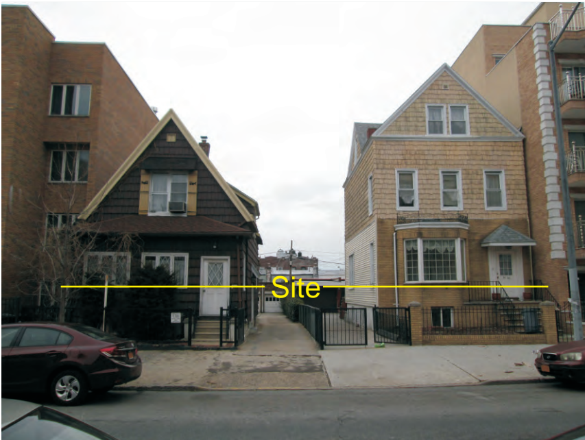
3. View of the Site, facing west.
