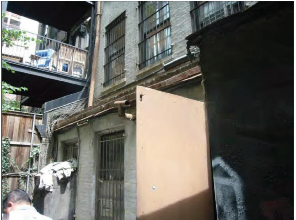
One-story build out on the south façade 3
