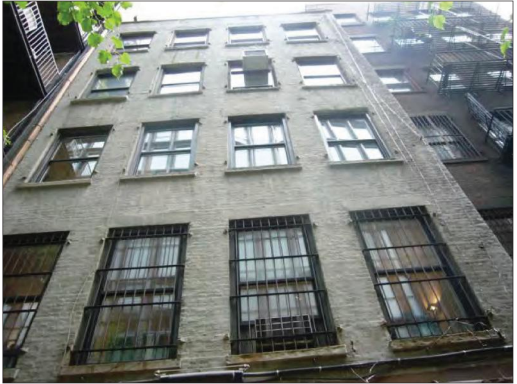
South façade of 41 Great Jones Street 2
