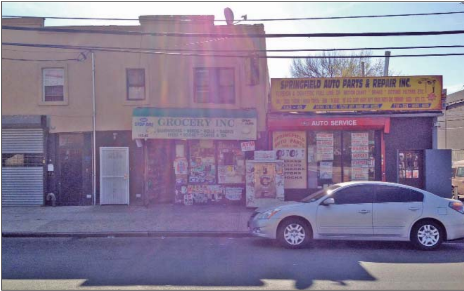
5. Existing mixed-uses on Springfield Boulevard, north of the applicant's commercial property.
