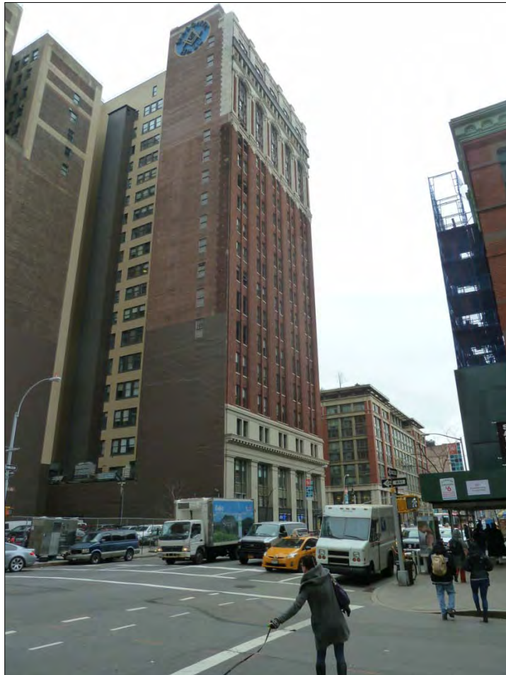
3. The Masonic Building at the corner of Sixth Avenue and W. 23rd Street in the Northern Sub-Area.
