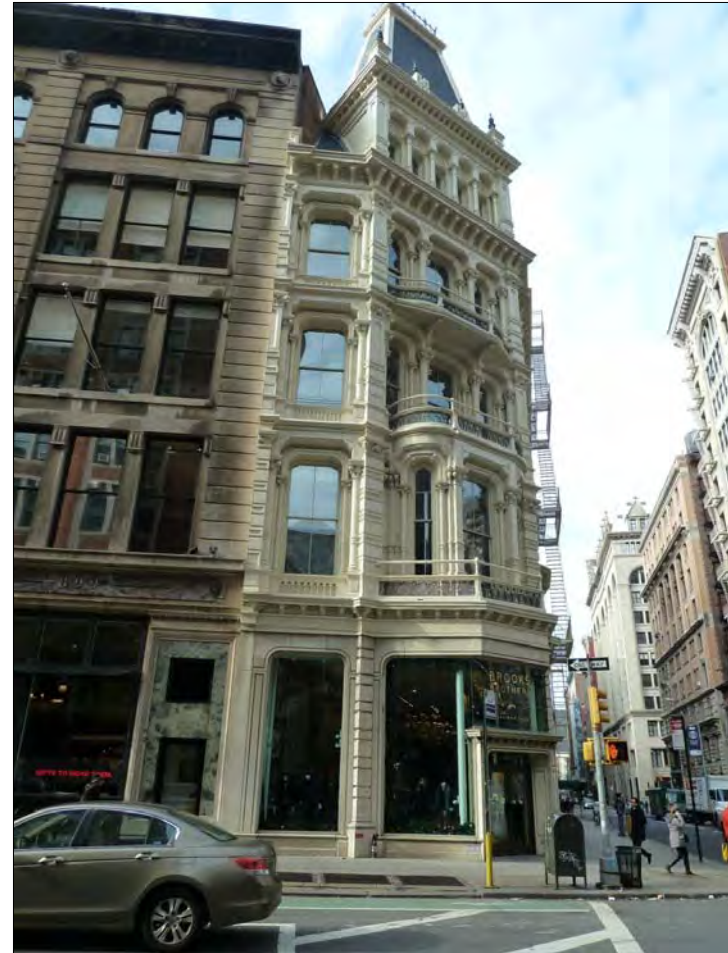
12. The former Lord & Taylor Building on the corner of W. 20th Street and Broadway; a remnant of the Ladies' Mile section of Broadway.
