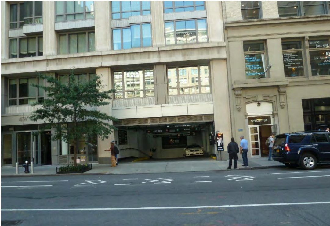
5: View from Project Site looking south on W 21st Street
