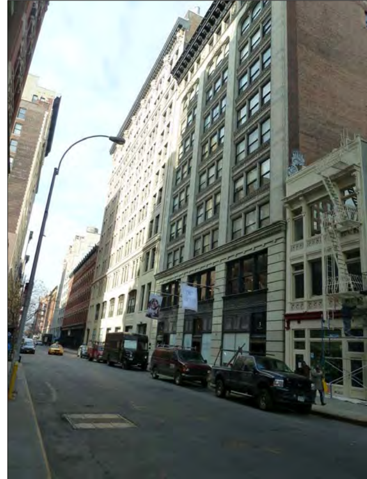
18. A typical view of buildings in the Northern Sub-area.
