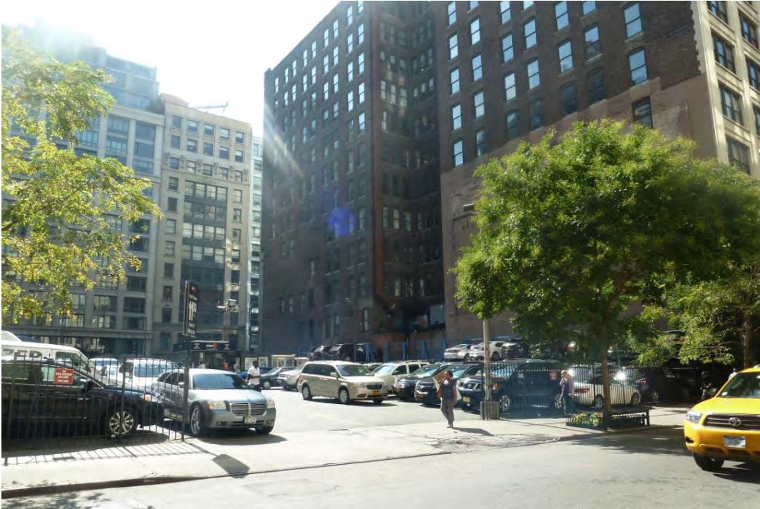
7: View of Project Site looking southwest from W 22nd Street
