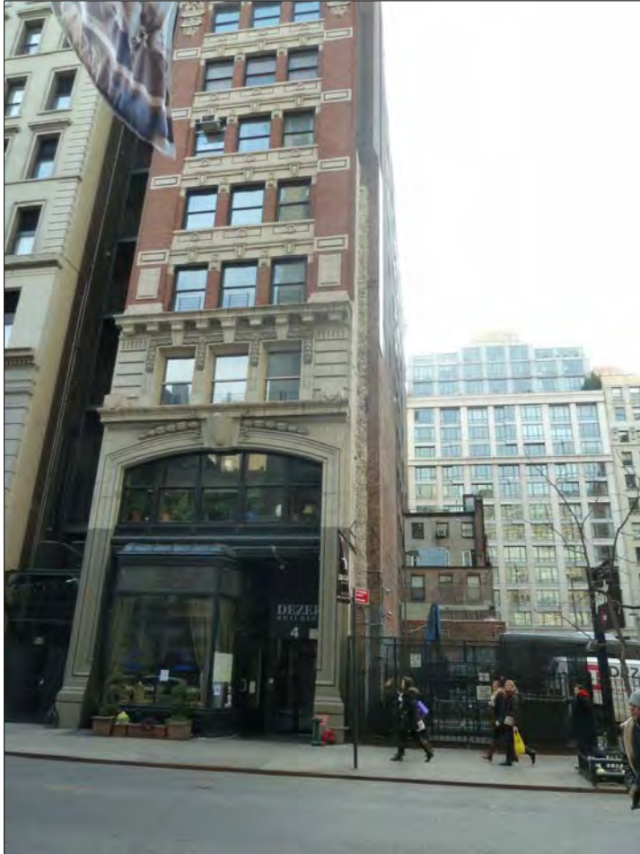
17. The Beaux-Arts style Dezer building located to the east of the project site on the W. 22nd Street frontage.
