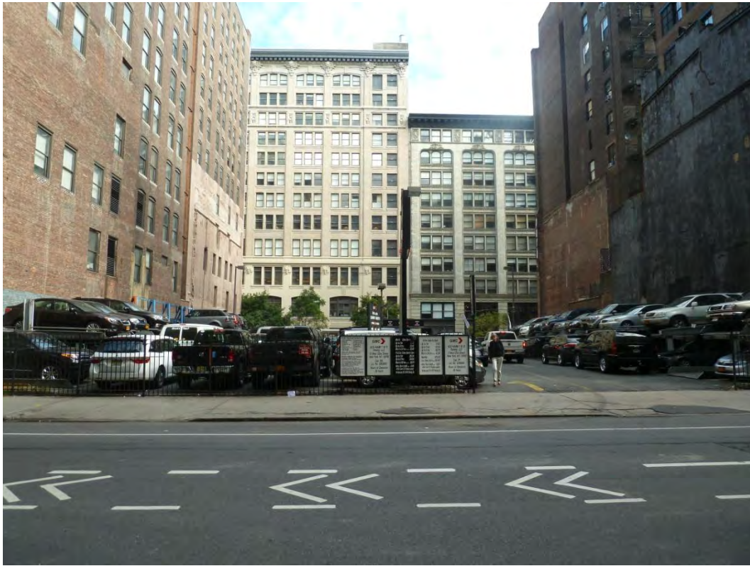
3: View of Project Site looking north from W 21st Street
