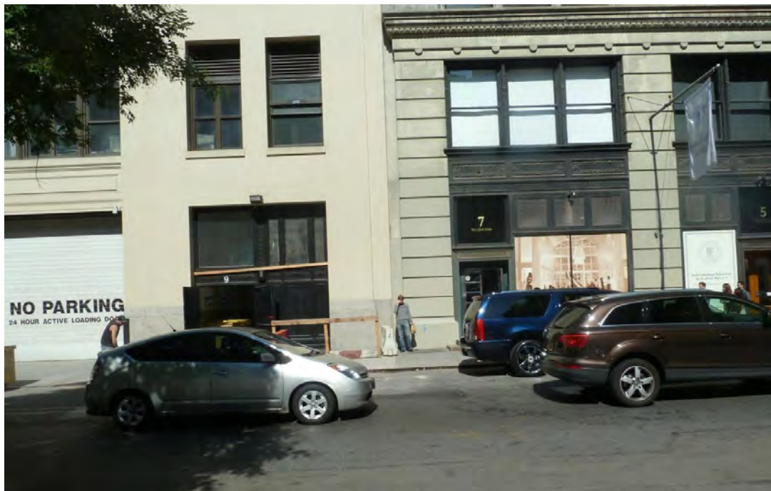
12: View from Project Site looking north on W 22nd Street
