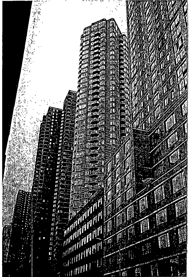
30 Looking east from 520 West 43 rd St.
