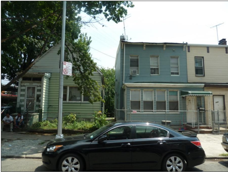
7. One and two family homes adjacent to Vaux Rd on 60 th St
