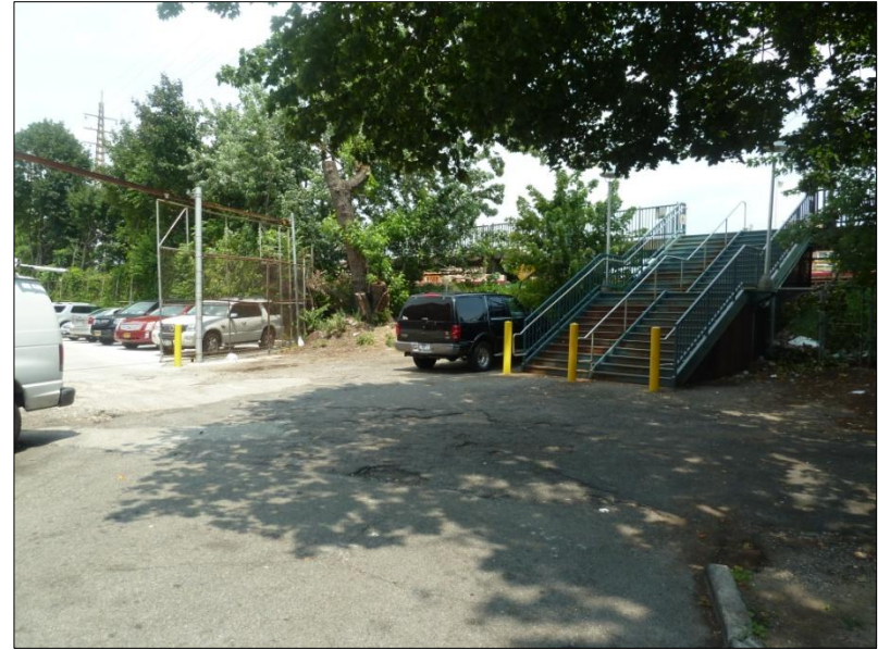
6. Stairs to Woodside LIRR station at Vaux Rd and 60 th St
