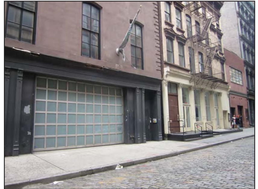
2. Project Site and adjacent lower-level retail spaces.
