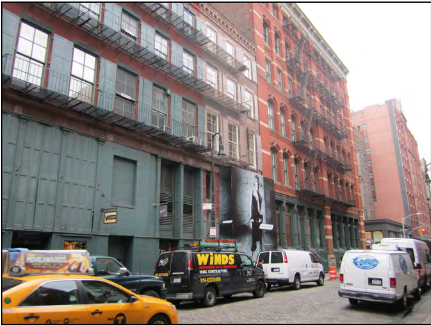
3. View south along east side of Mercer Street.
