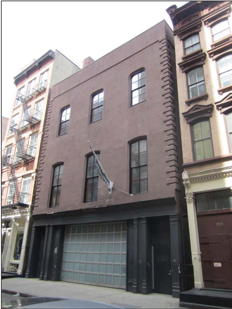
1. Existing front facade of 155 Mercer Street (Project Site).
