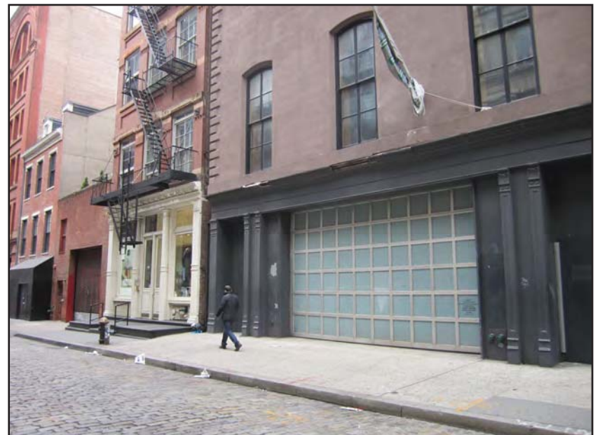
3. Project Site and adjacent lower-level retail spaces.
