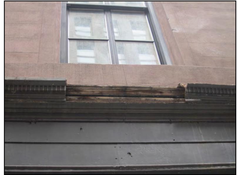
2. Missing portion of cornice beneath central second floor window.
