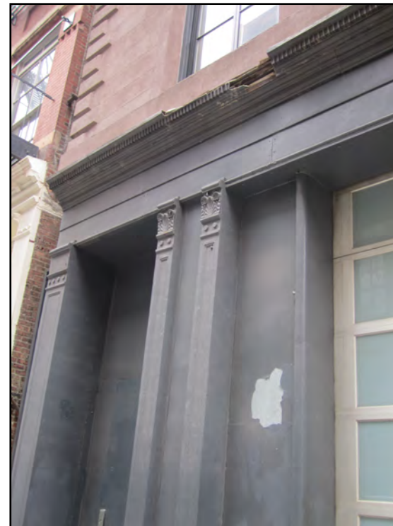
2. Missing portion of cornice beneath central second floor window.
