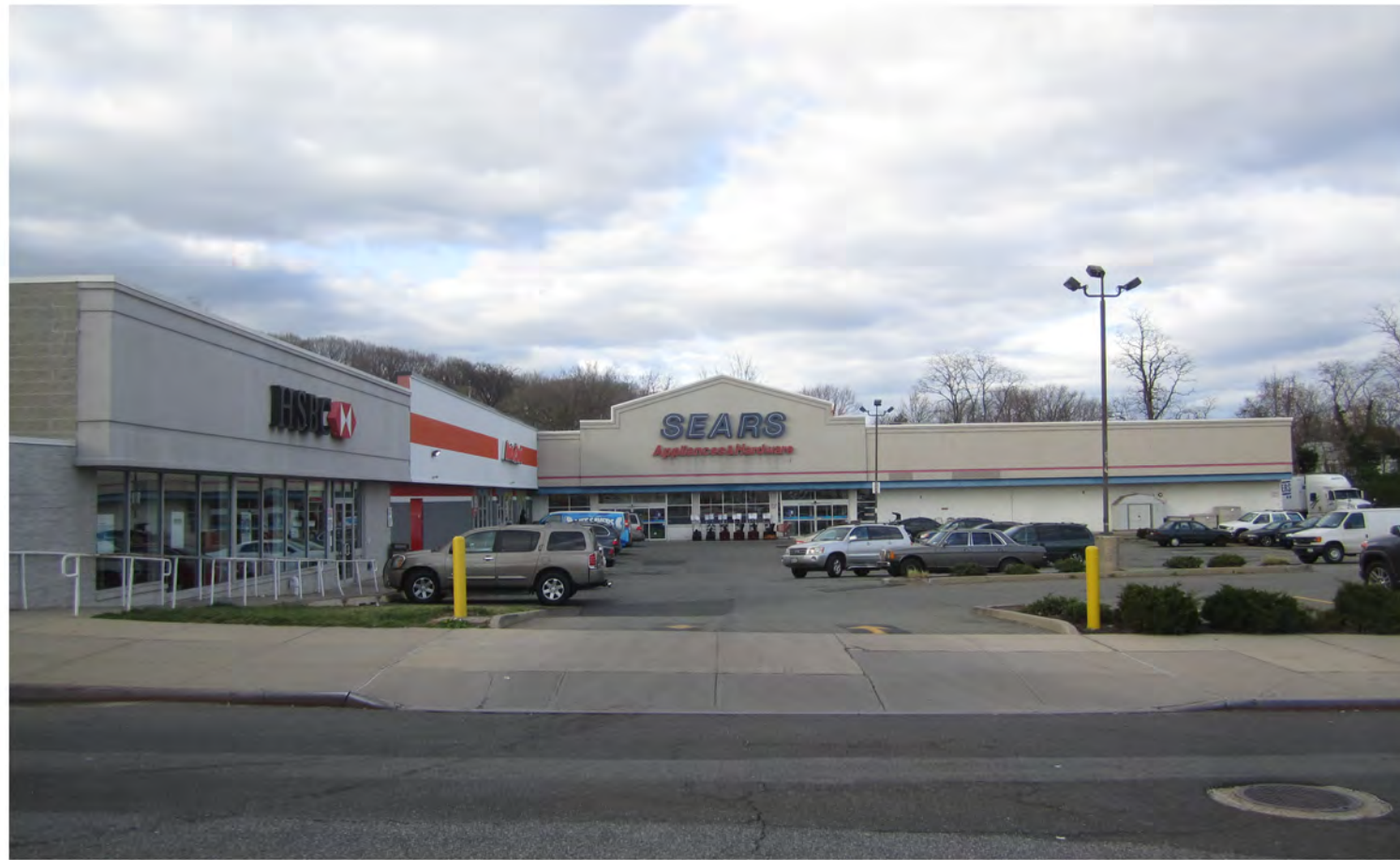
04 VIEW OF SITE FOM BRADDOCK AVENUE FACING NORTH
