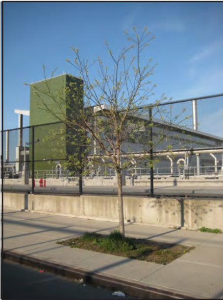
1. Street trees around Newtown Creek WWTP.
