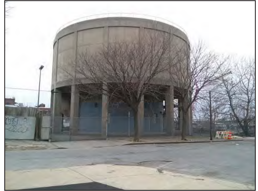
2. Existing sludge tank.
