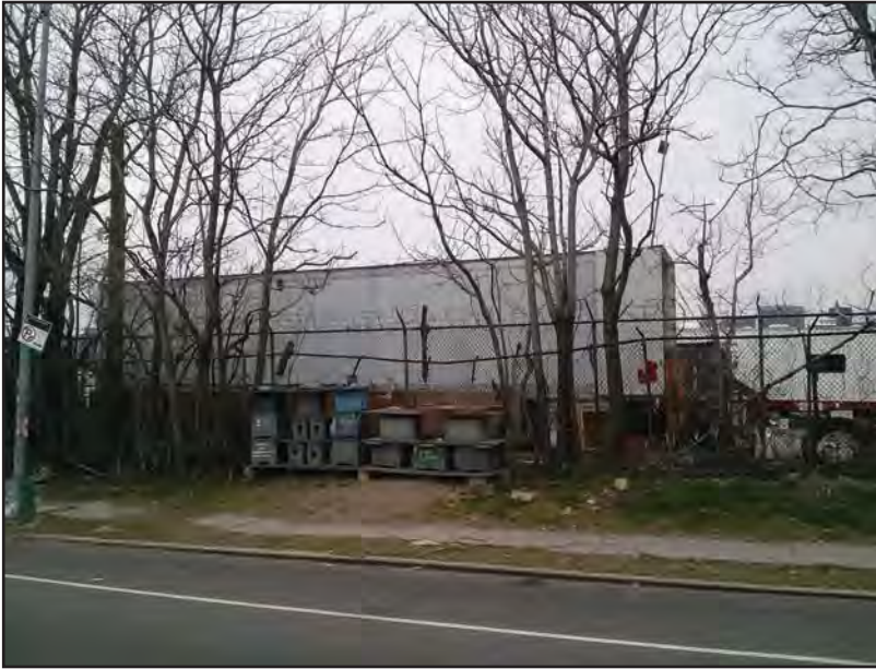
1. Poor sidewalk quality.
