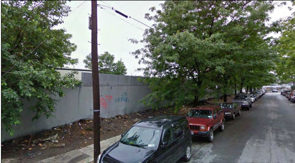
5: View of Projected Development Site 5 looking south from DuPont St.
