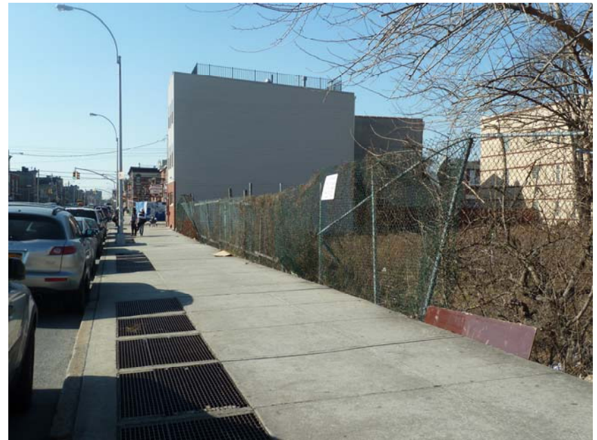
2 View of the development site's Pitkin Ave. frontage (looking west)
