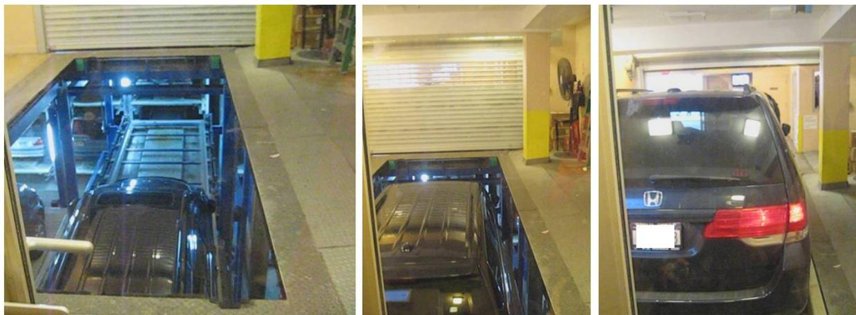
Figure 8 Automated vehicle retrieval in 123 Baxter facility
