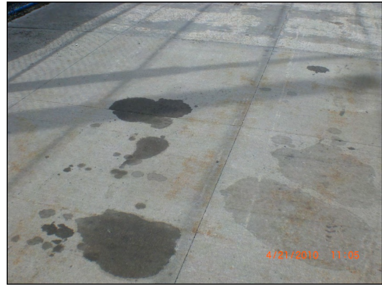
Photograph 6. Surface staining on the northern Property sidewalk near the entrance to the athletic field.
