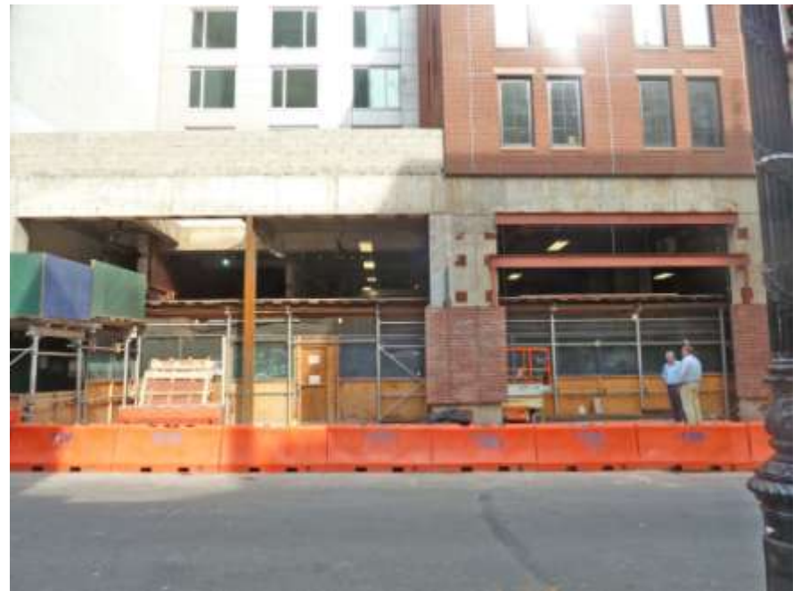
2 Project site frontage on the east side of Orchard Street.
