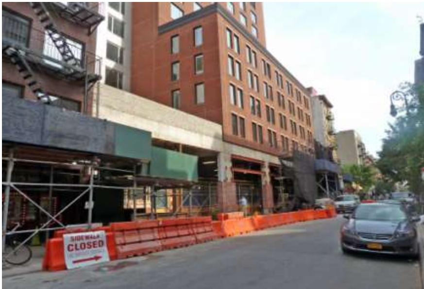
3 Street view looking south at the project site on Orchard Street.
