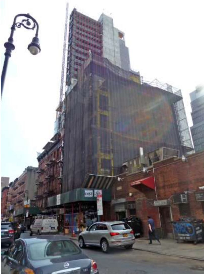
5 Street view looking south on Ludlow Street at the project site.
