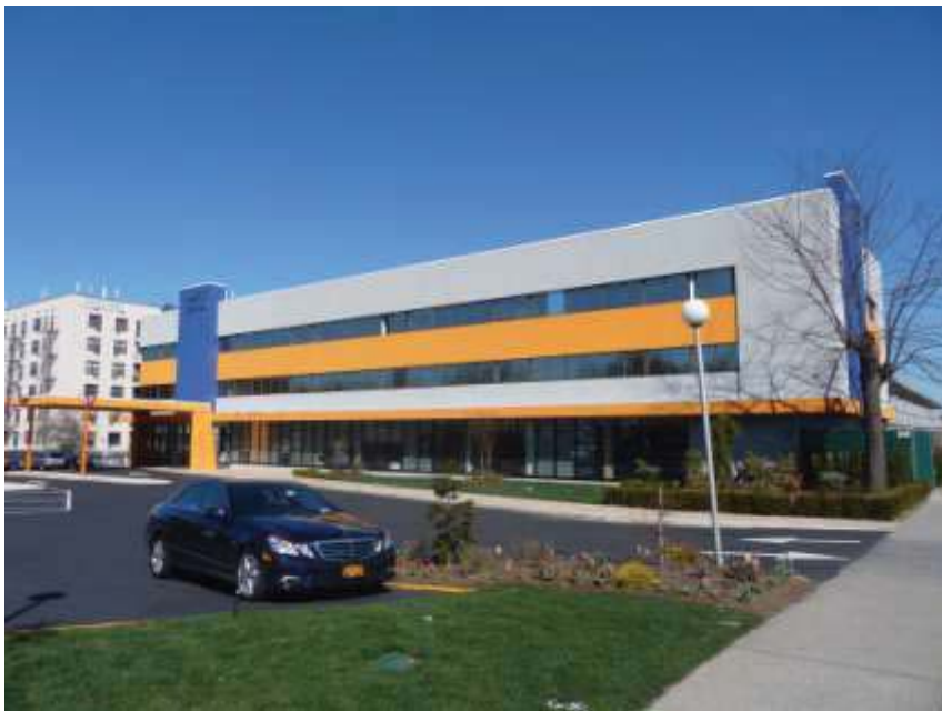
7 The Brooklyn Amity School to the southwest of the Project Site.
