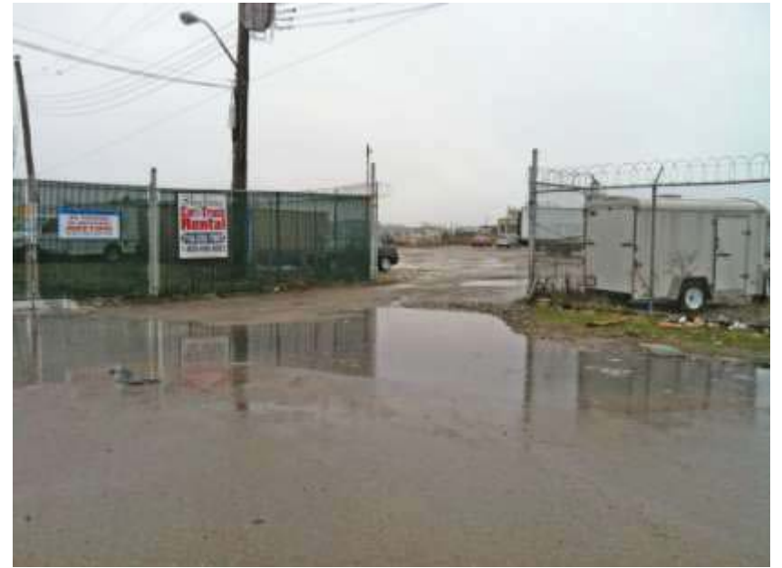
4 Entrance to the Project Site on Voorhies Avenue.
