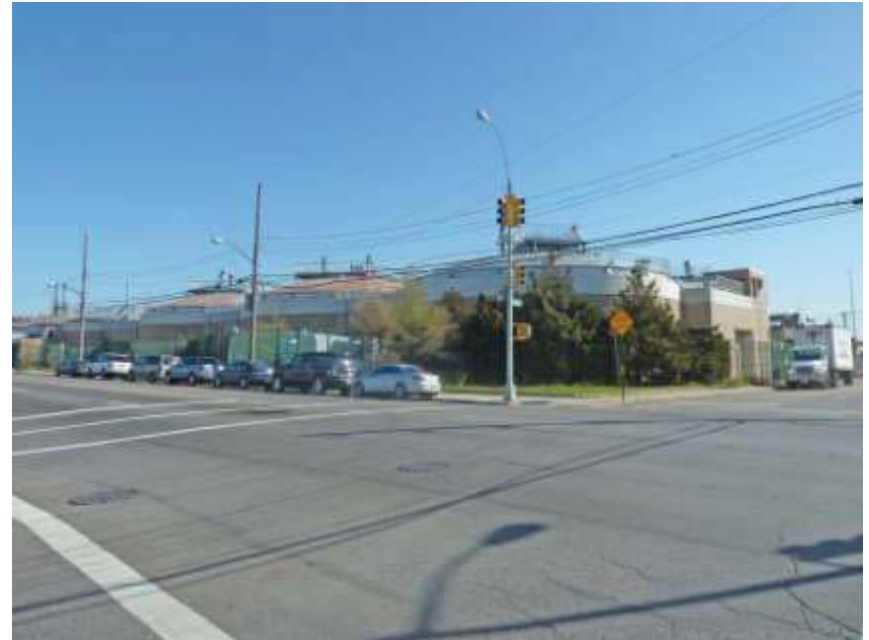
6 The Coney Island Wastewater Treatment Plant, northwest of the Project Site across Voorhies Avenue.
