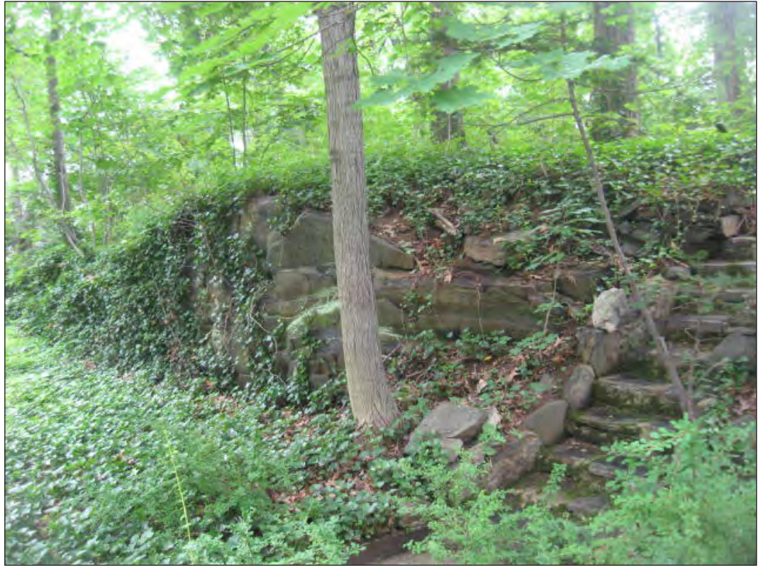
View of outcrop located on the northwestern side of the Project Site along the Fieldston Road sidewalk 3
