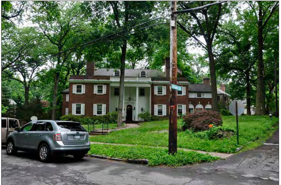
4710 Fieldston Avenue/401 Indian Road 9
