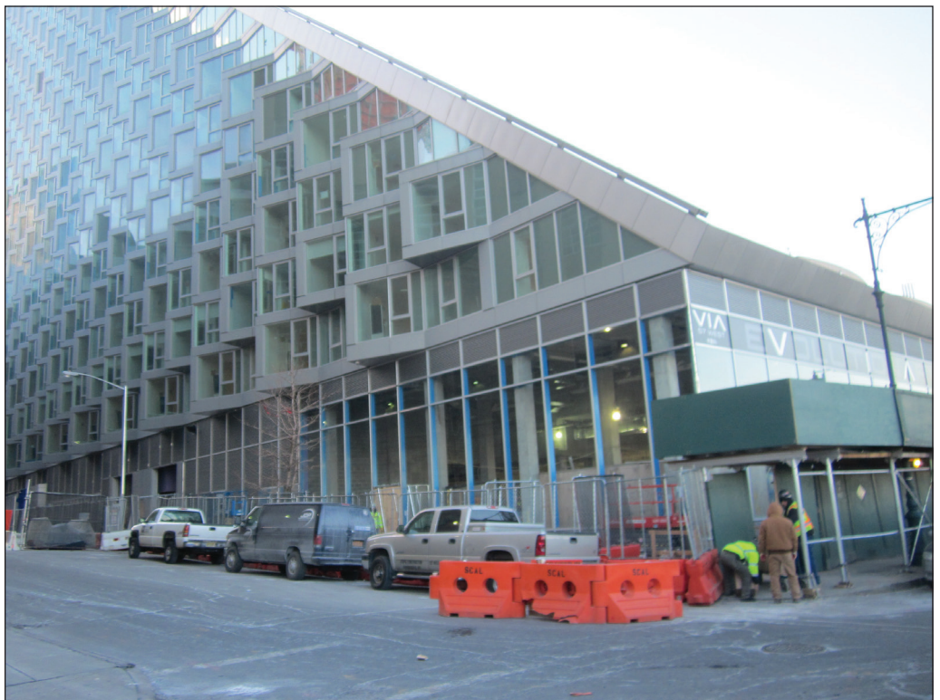
View of the Development Site from West 58th Street facing southeast 4
