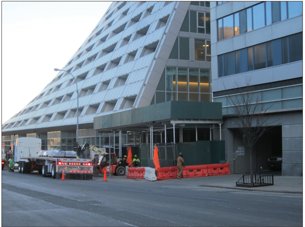
View of the Development Site from West 57th Street facing northwest 2
