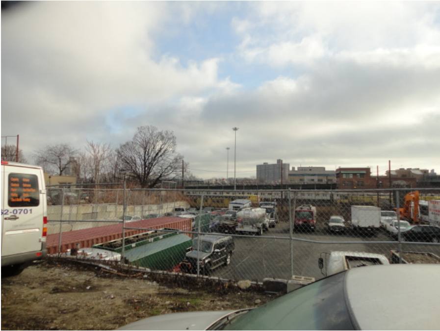
Photo 3. View East of NYCT Maintenance Yard
