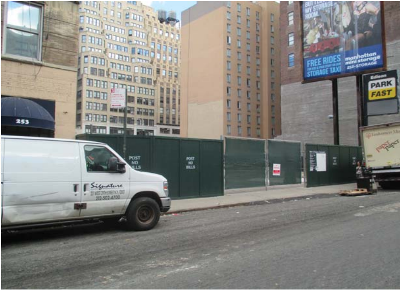
9- View from West 28th Street looking northeast towards Development Site
