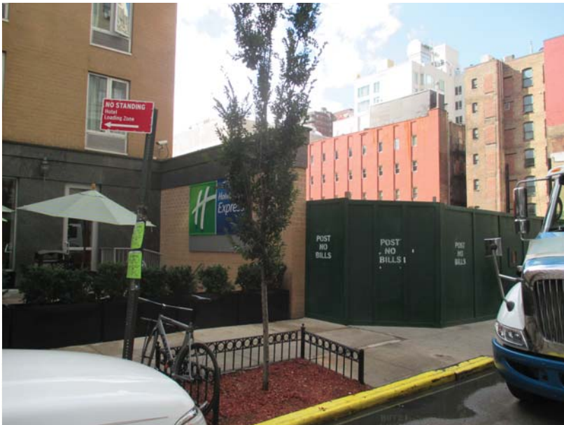
3- View from West 29th Street looking south towards Development Site
