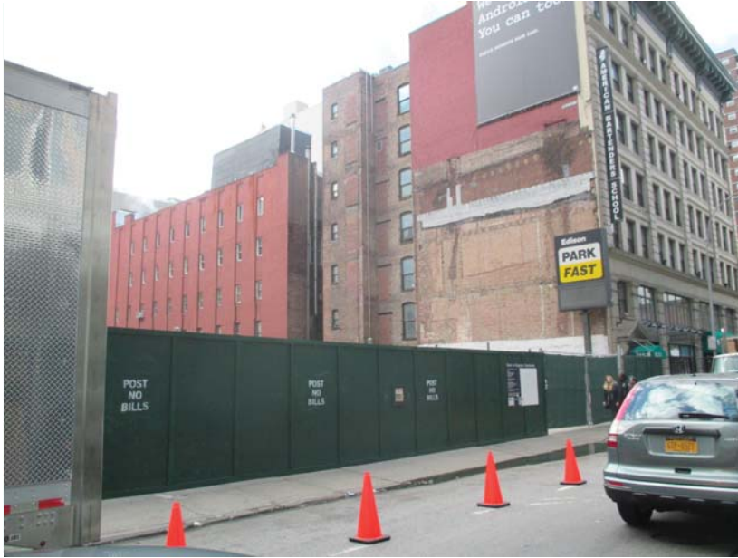
1- View from West 29th Street looking southwest towards Development Site
