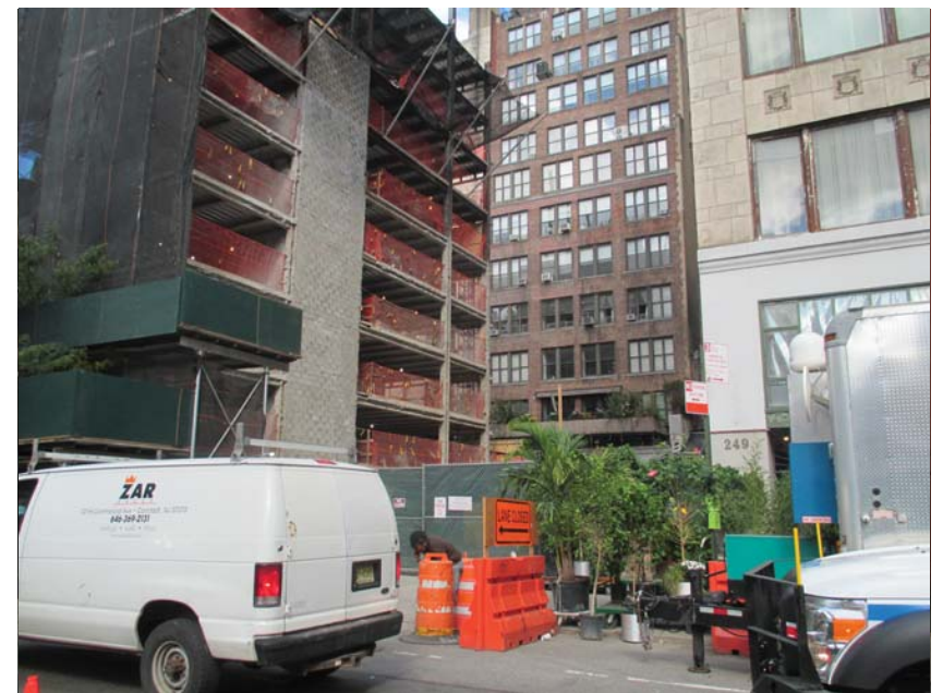
8- View from West 29th Street looking north
