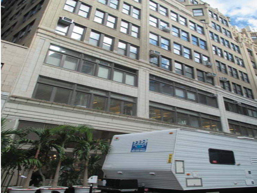
5- View from West 29th Street looking north
