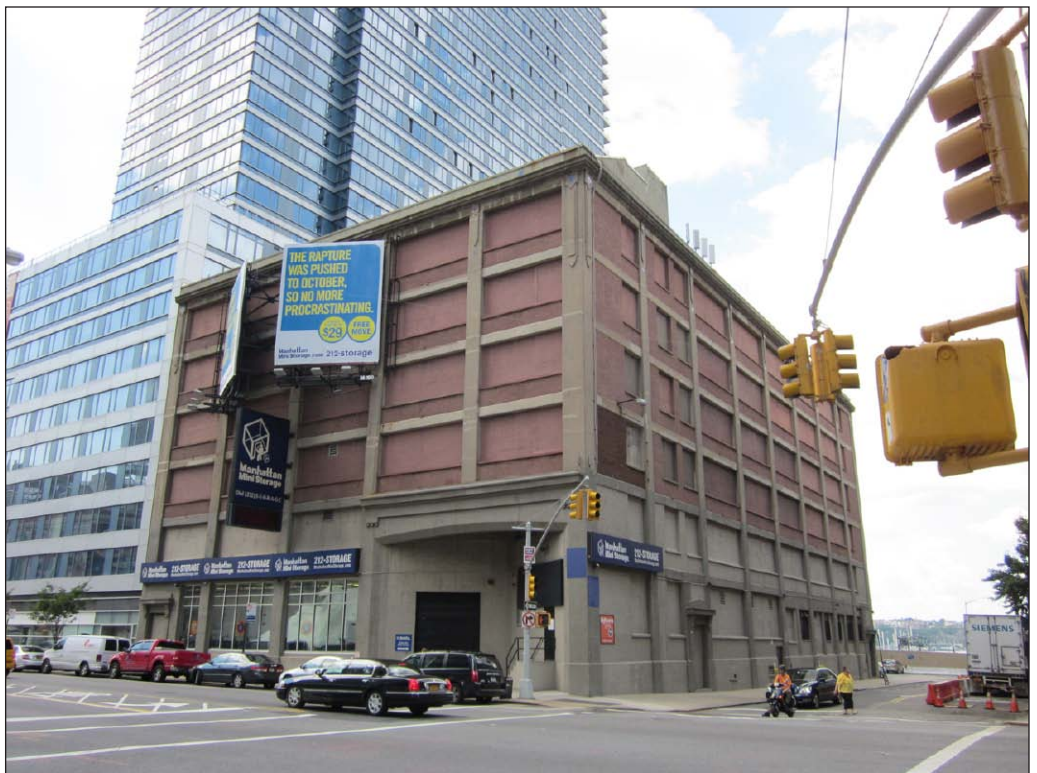
Projected Development Site 2, view southwest from West 58th Street and Eleventh Avenue 2
