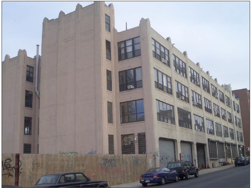
Former Rokeach & Sons Warehouse, 63-81 North 3rd Street 14
