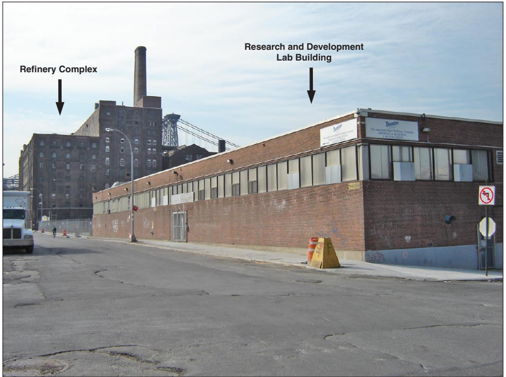
View southwest on Kent Avenue 6
