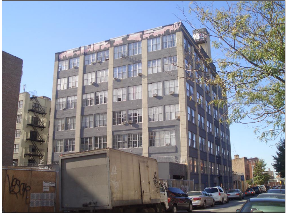
Former Gretsch Building #2 22 164-114 South 4th Street
