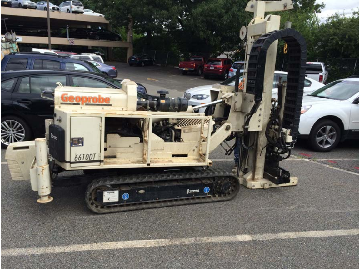
Photograph No. 1: Installation of soil boring VHB-2 utilizing a Geoprobe® hydraulic push drill rig.
