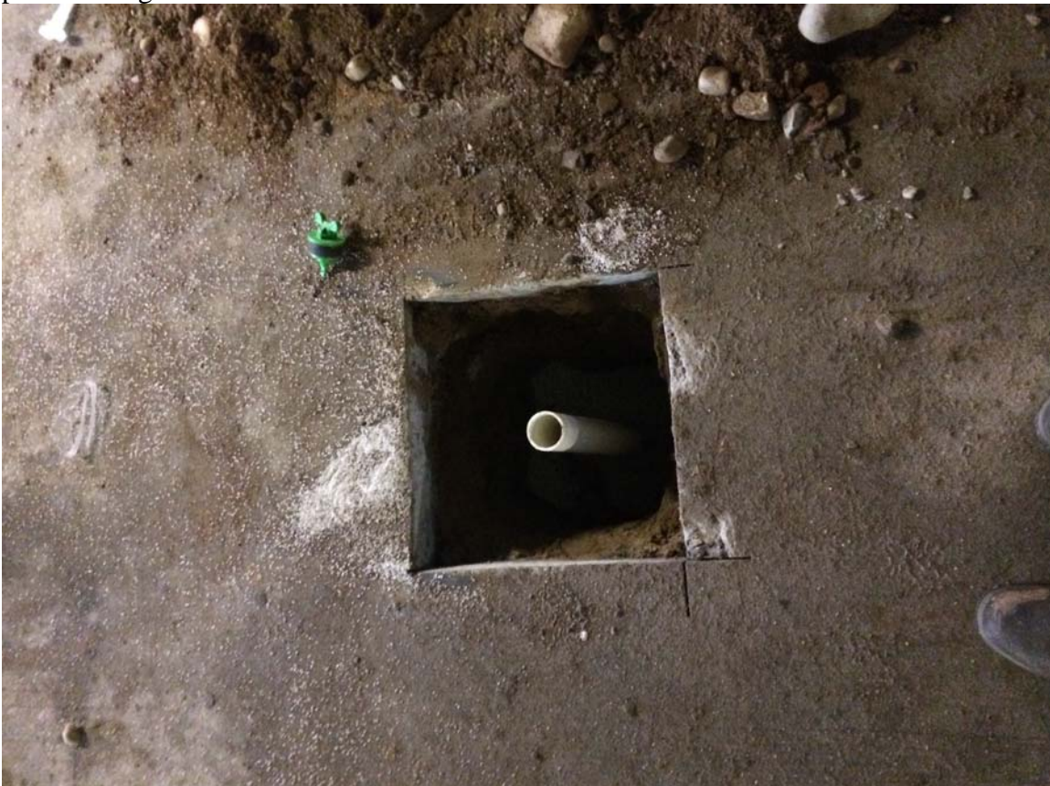
Photograph No. 2: Installation of monitoring well MW-2.
