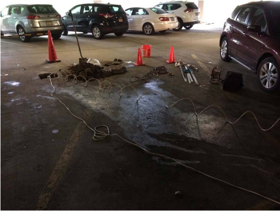
Photograph No. 3: Development of monitoring well MW-1 utilizing a groundwater whale pump.
