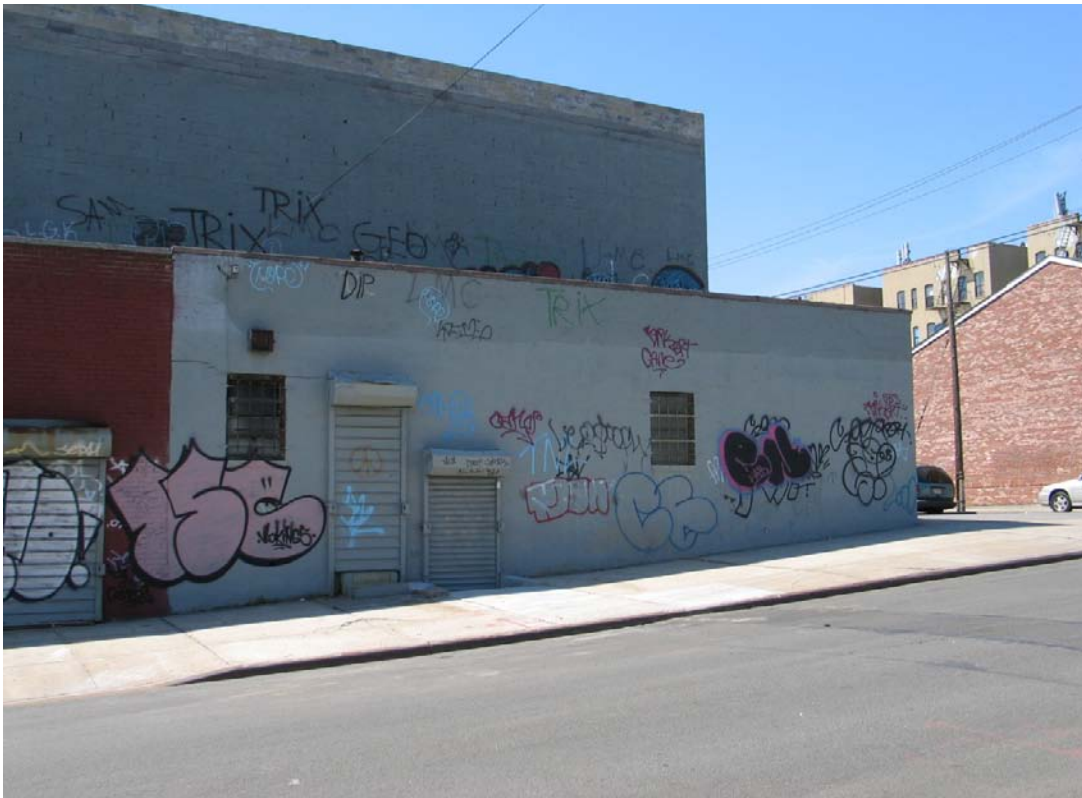
Photograph 11: Block 3013, Lot 35, facing southwest from East 172nd Street.
